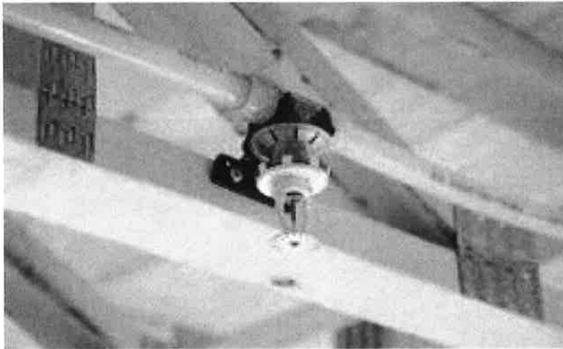
Photos & Drawings 12: A common residential sprinkler installation
