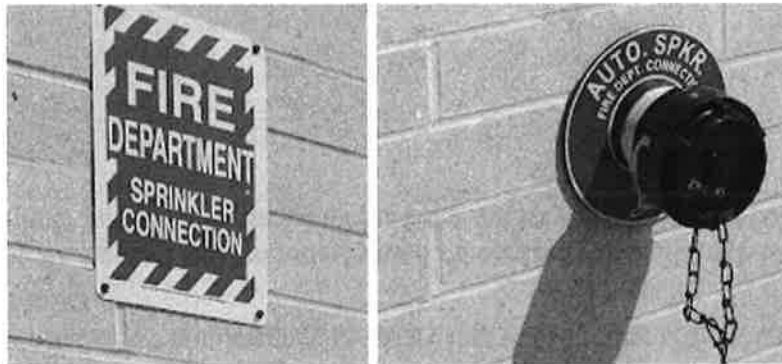
Photos & Drawings 11: Sprinkler location sign and FD connection
