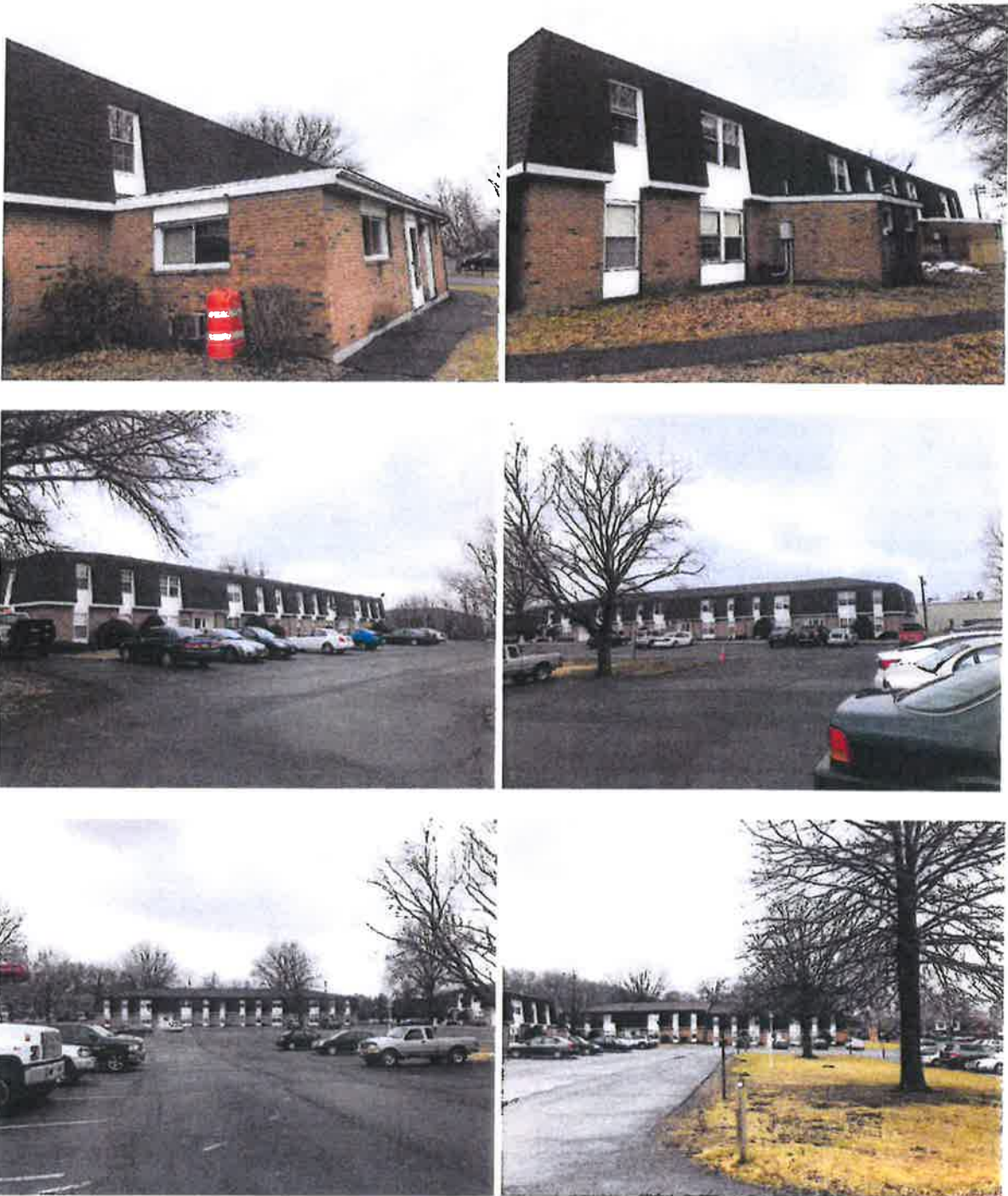
Typical exterior views of the subject complex
