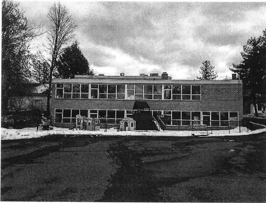
Figure 13: Eastward view of Temple Emanuel's west face with windows and playground representing the educational side of the structure. Photograph by Ethan Dickerman, HPA, 2024.
