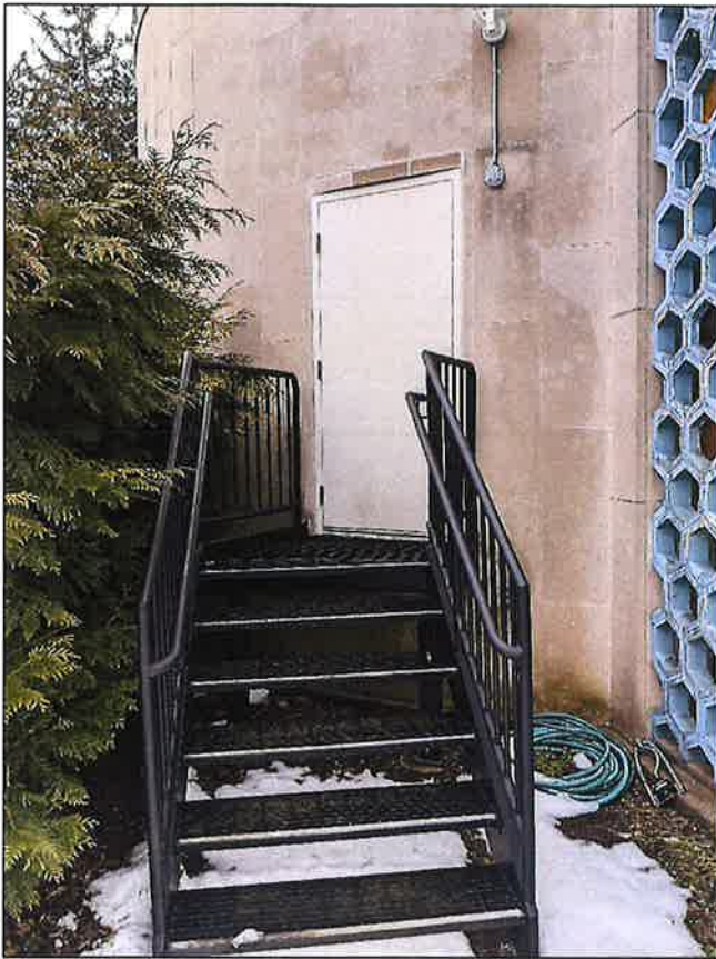
Left, Figure 15: Image of fire exit installed on the eastern (Albany Ave) face following the 2003-5 renovations and which is screened by shrubbery. Photography by Ethan Dickerman, HPA, 2024. Right, Figure 16: Close-up photograph of blue hexagonal breezeblock screen highlighting varies degrees of decay. Photography by Ethan Dickerman, HPA, 2024.
