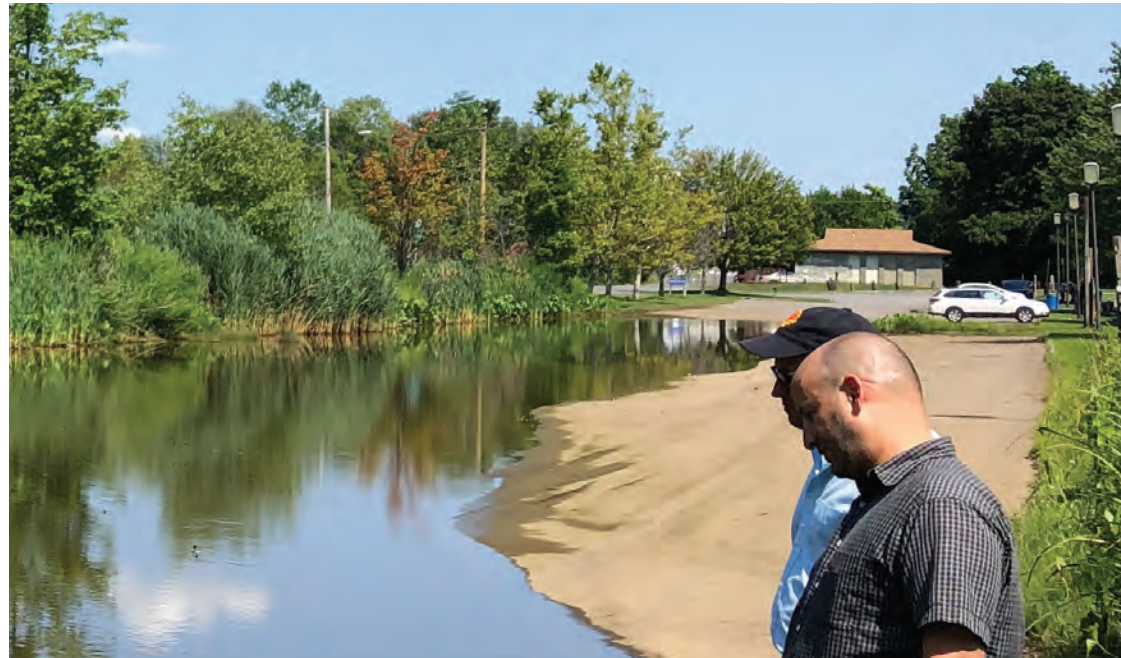
Existing Parking Lot Area
