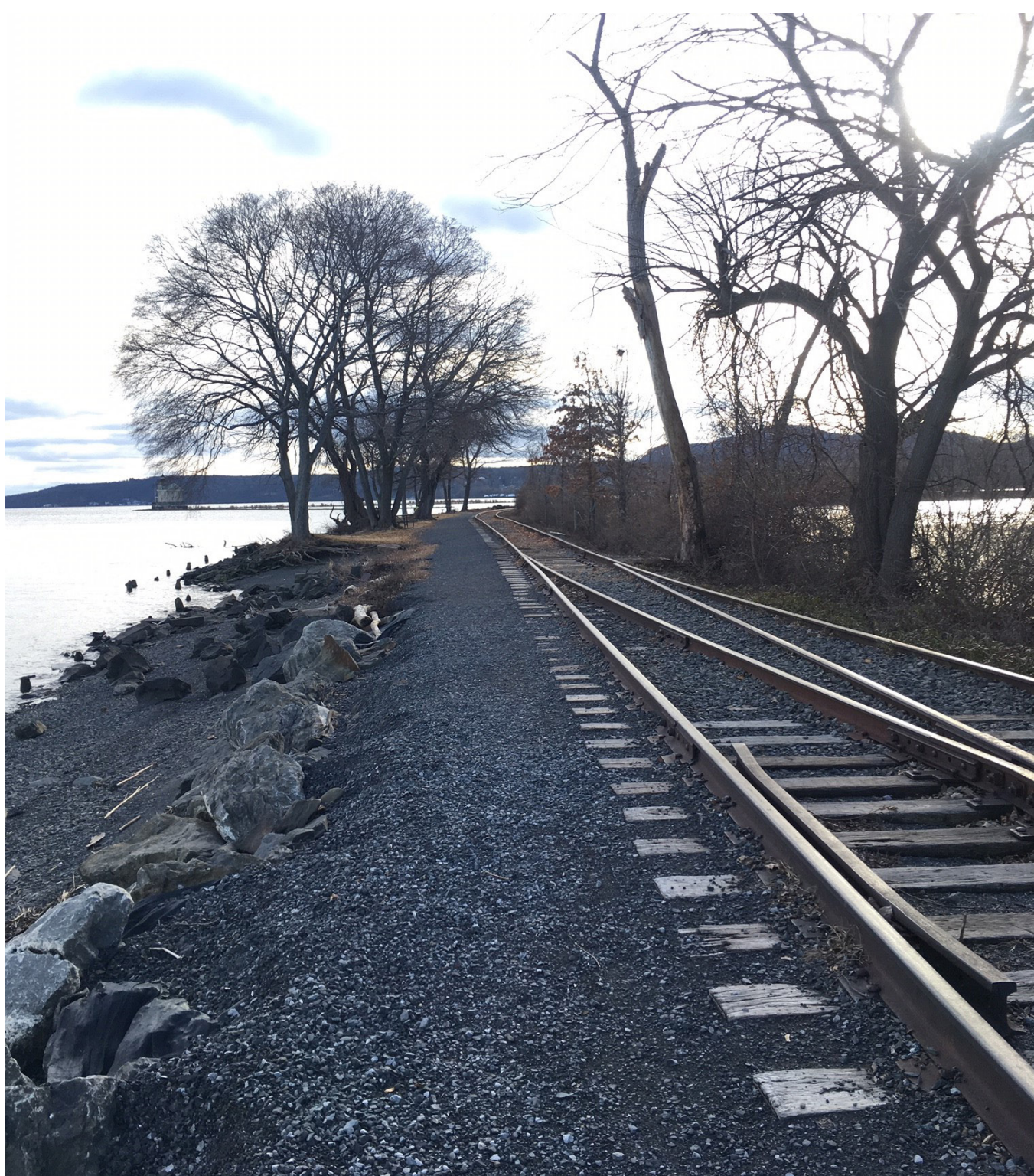
Site photos of existing conditions taken in January 2019
