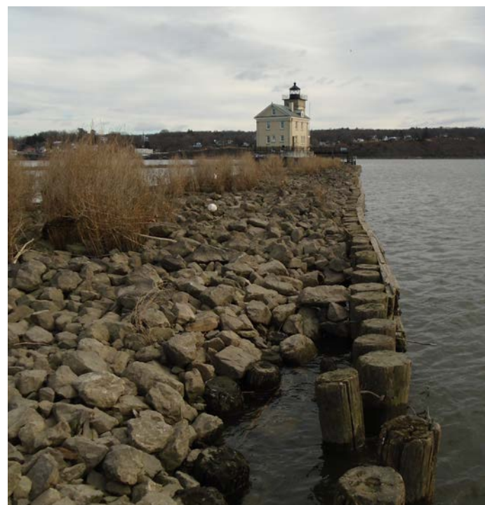
Erosion along the jetty, observed in January 2019
