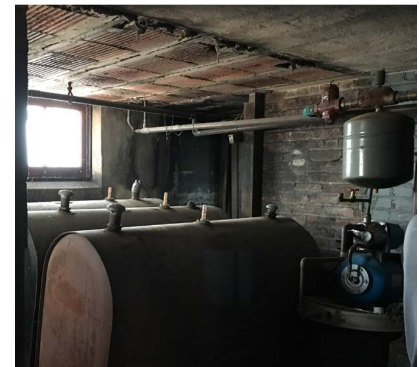
The lighthouse basement, which lacks utility connections
