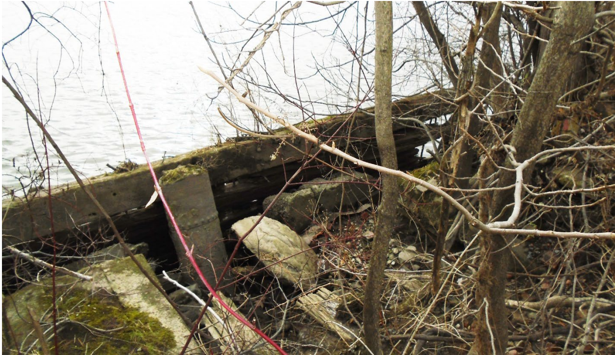
Figure 12: An Example of Scoured Earth Behind Stabilization Infrastructure Found in the Project Area
