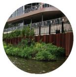
Sheet piles walls can incorporate elevated walkways, kayak tie-up areas, floating wetlands, and incremental attachment points to accomodate sea level rise.
