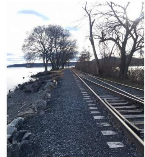
Site photos of existing conditions taken in January 2019
