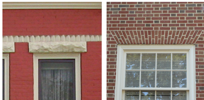
Figure 405.14.E.2.a Headers. Stone Lintel (left) and Brick Jack Arch (right)
