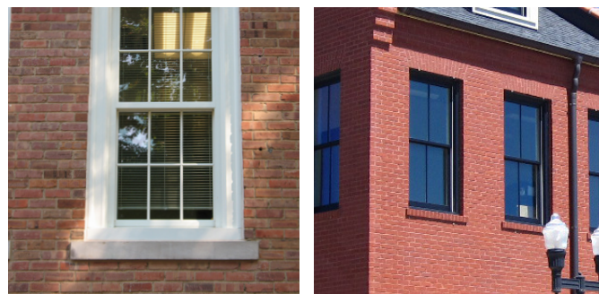
Figure 405.14.E.2.b: Sills. Cast Concrete (left) and Brick (right)
