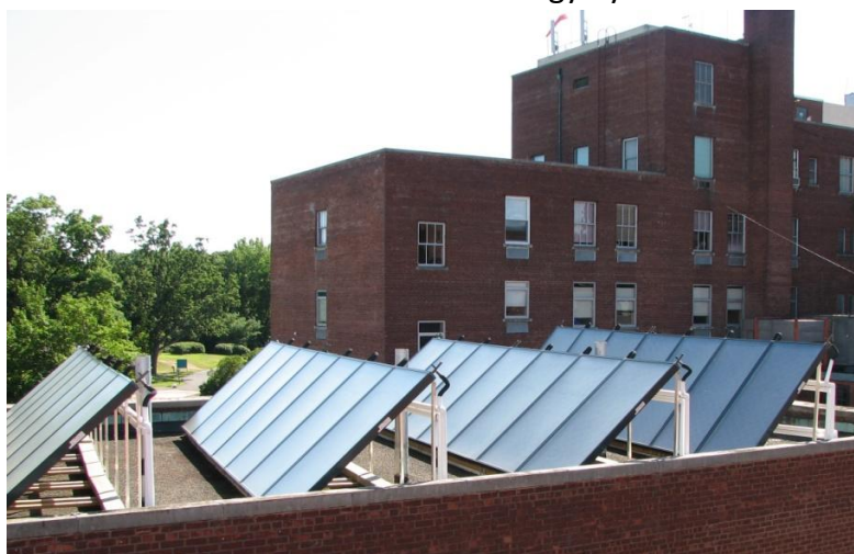
Solar Thermal Hot Water System
