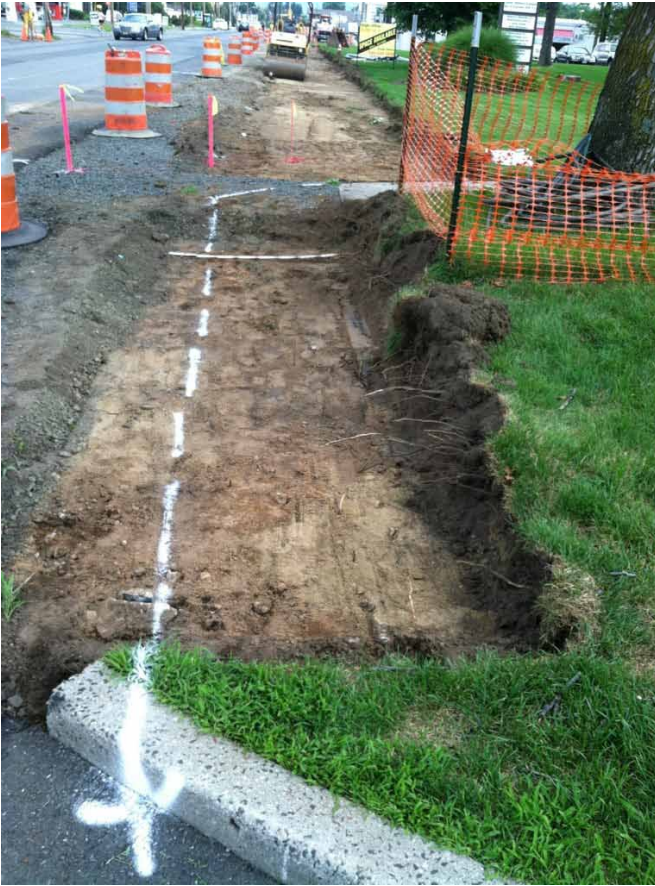
Figure 36. Protecting existing trees appropriately when doing needed construction. Utilization of structural soil for street tree plantings along sidewalks and other paved areas allows installation of hardscape features such as concrete or bluestone walks and granite curbs without damage from healthy tree root growth. Underneath the tree in the image below is a large bed of CU™ Structural Soil extending several feet in either direction around and below the root ball.
