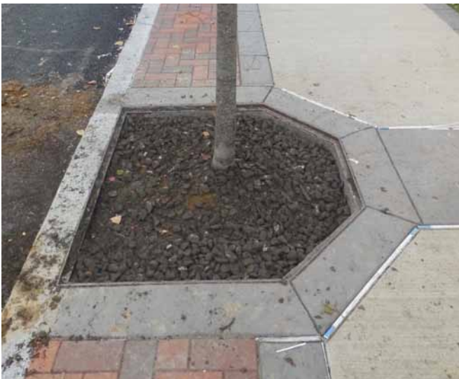
Figure 36. Protecting existing trees appropriately when doing needed construction. Utilization of structural soil for street tree plantings along sidewalks and other paved areas allows installation of hardscape features such as concrete or bluestone walks and granite curbs without damage from healthy tree root growth. Underneath the tree in the image below is a large bed of CU™ Structural Soil extending several feet in either direction around and below the root ball.
