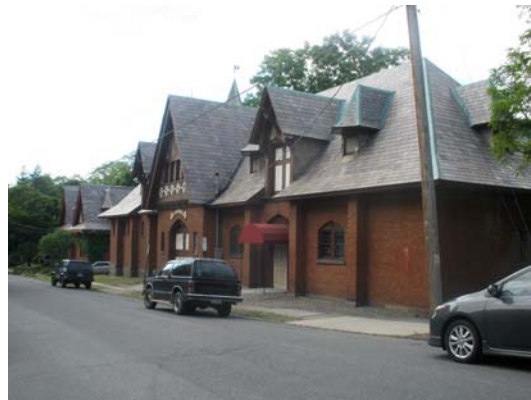
The Coykendall carriage houses on Augusta Street
