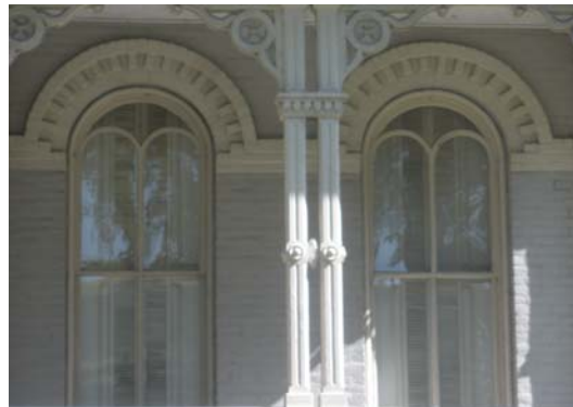
Porch and window details at 18-24 Stuyvesant
