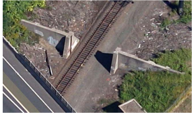
Figure 7: Photograph of Typical Bulkhead Installation
