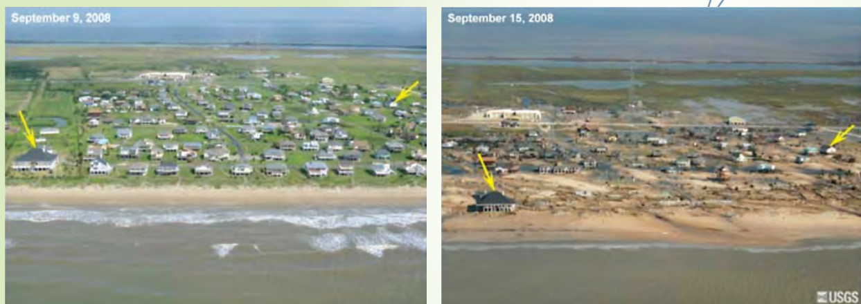
FIGURE 4: Shoreline Before and After Hurricane Ike (Galveston, Texas)
