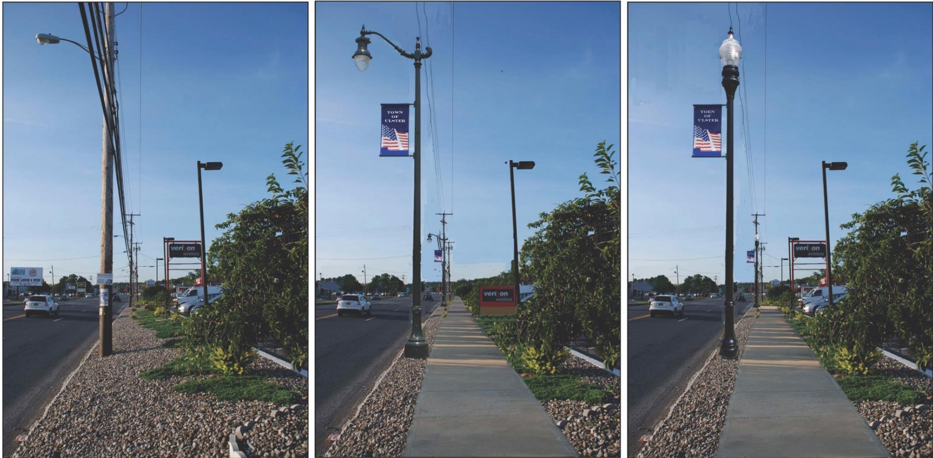
Above (Left to Right): View of existing conditions on U.S. Route 9W corridor looking north from Kings Mall on east side of U.S. Route 9W; same view showing new period streetlights with banners, a new sidewalk, relocation of telephone and cable lines (see Appendix A) replacement of Verizon pole sign with monument sign and removal of billboard and pole signs on left side of photo; and same view with new period lighting with banner with the Verizon pole sign, but billboard on left side of photo removed. These illustrations show how streetlights, sidewalks and sign regulation affect the appearance of the corridor.
