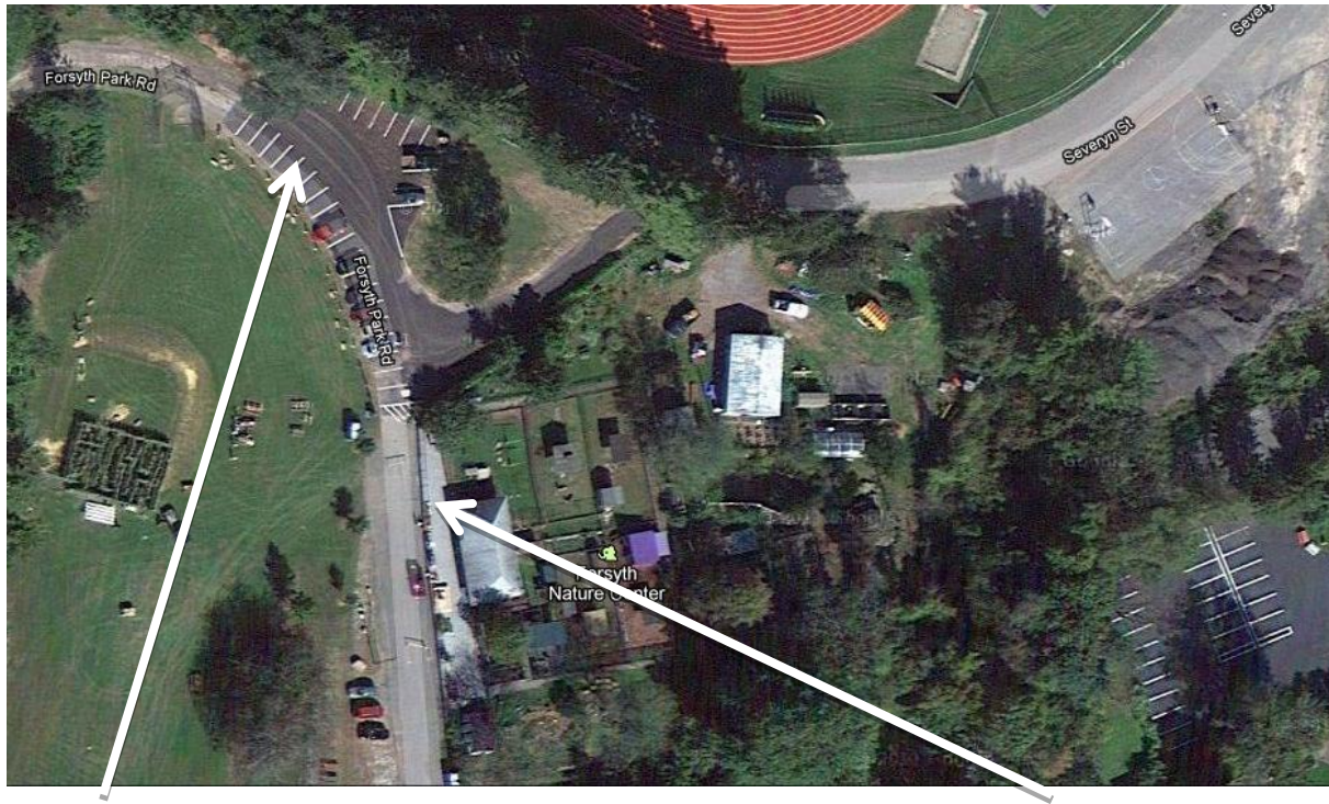
Porous Asphalt Parking Lot at Forsyth Nature Center
