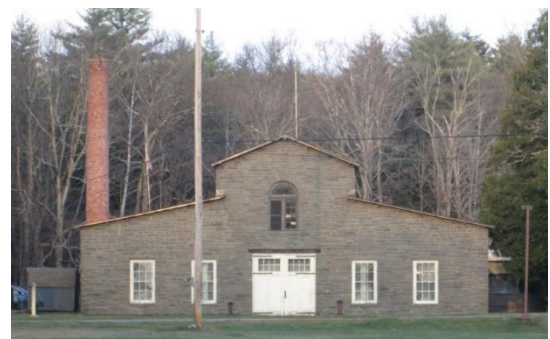
Edmund T. Cloonan Water Treatment Plant
