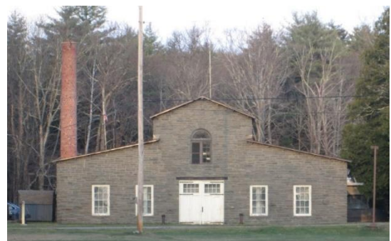
Edmund T. Cloonan Water Treatment Plant
