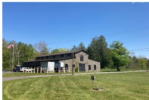
Edmund T. Cloonan Water Treatment Plant
