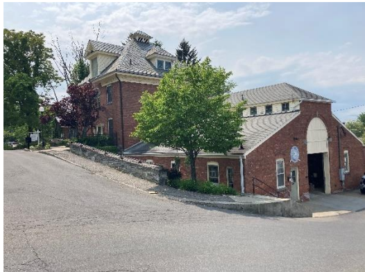
111 Jansen Ave Building
