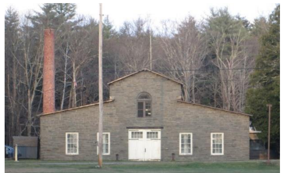
Edmund T. Cloonan Water Treatment Plant
