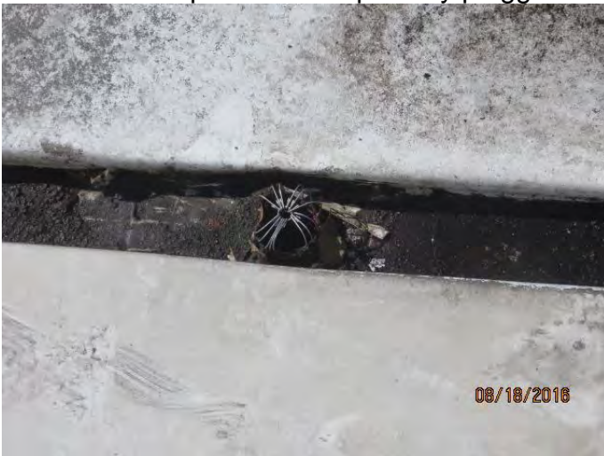
Photo 4 downspout strainer partially plugged
