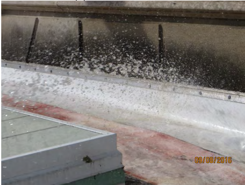
Photo 13 Close up photo 12
