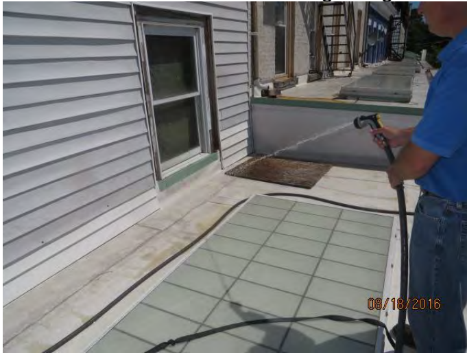
Photo 23 water test base flashing along base of wall over reported leak locations
