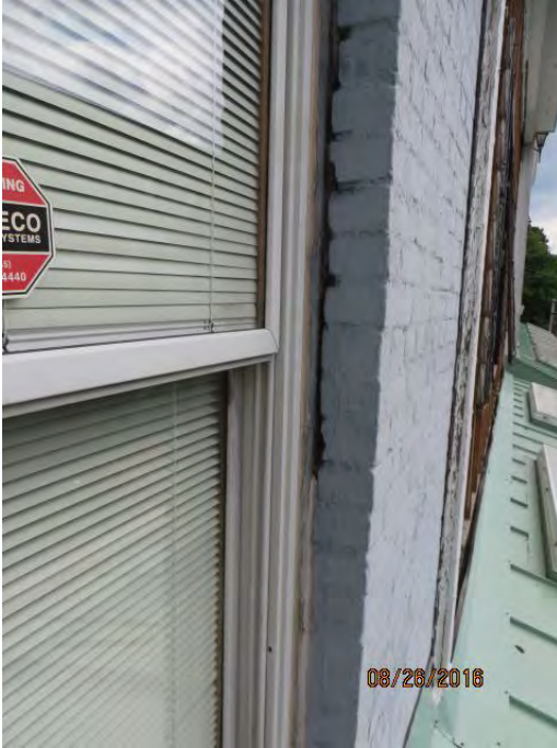
Photo 12 Opening between window jamb frame and brick wall
