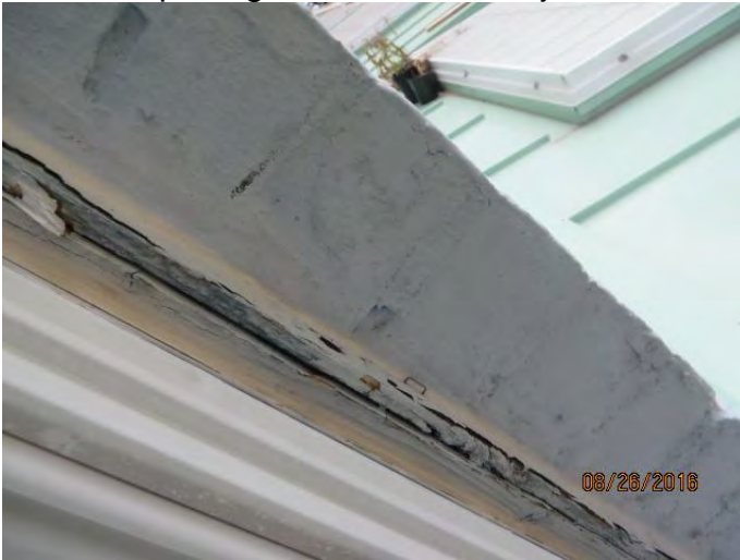
Photo 9 Opening between window jamb frame and brick wall
