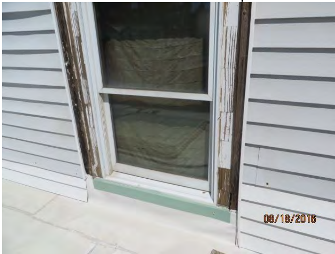
Photo 10 window above area of reported leaks
