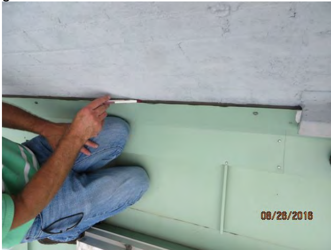
Photo 18 Sealant at top of green metal base flashing cracked and not adhered to green metal
