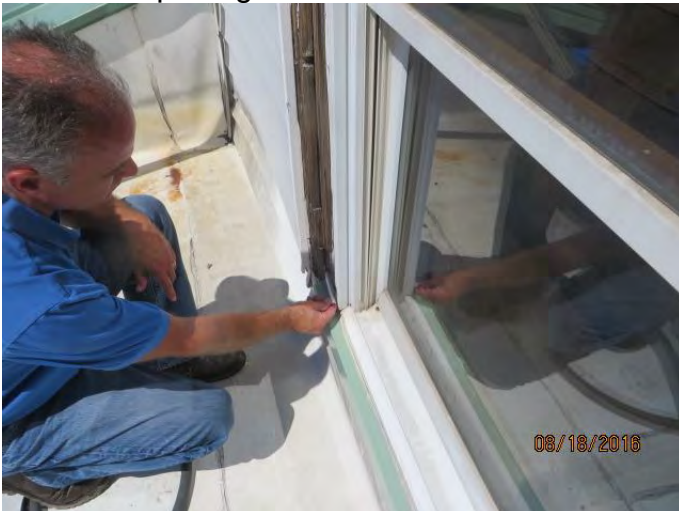
Photo 21 opening in window frame
