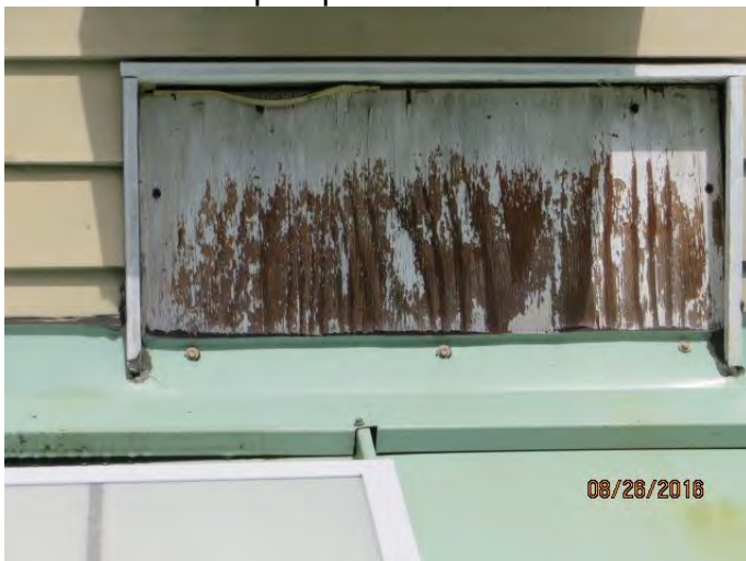
Photo 6 Close up of photo 5
