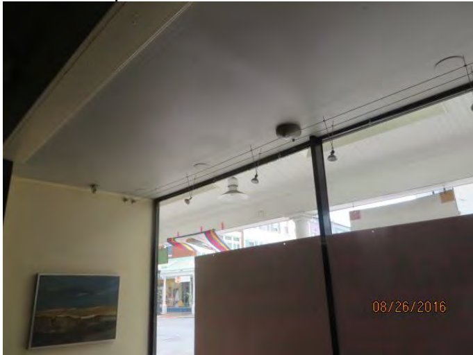
Photo 2 Reported leaks on interior surface of front display window
