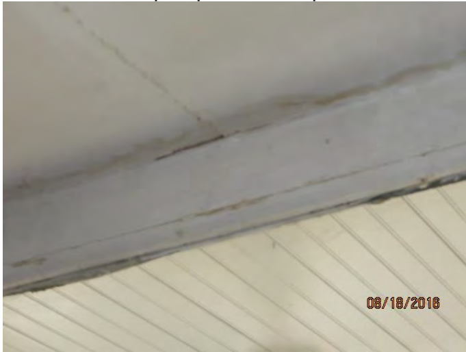
Photo 4 close up of photos 3, reported area of leaks after heavy blowing rain
