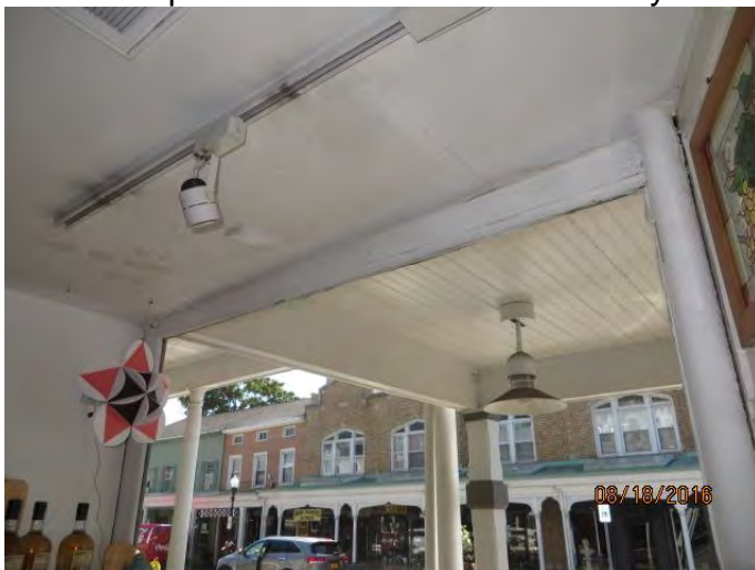
Photo 3 reported area of leaks after heavy blowing rain
