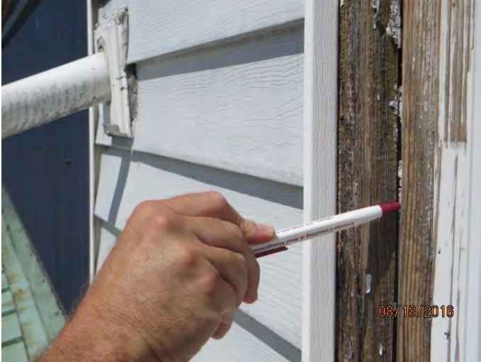
Photo 19 cracks in window frame
