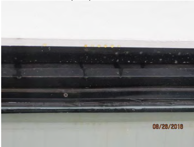
Photo 15 Close up of photo 14
