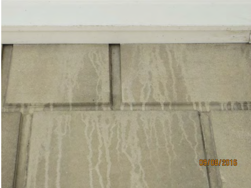
Photo 11 Water stains on wall beneath canopy, previously not reported
