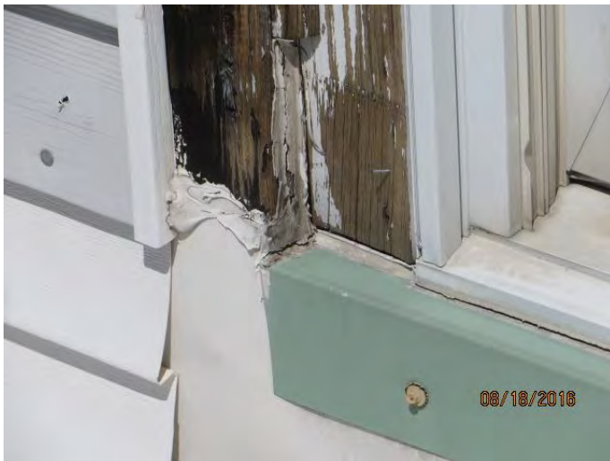
Photo 11 cracks in window frame
