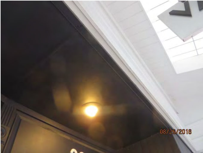
Photo 21 Water leak at vestibule at 11:17 AM
