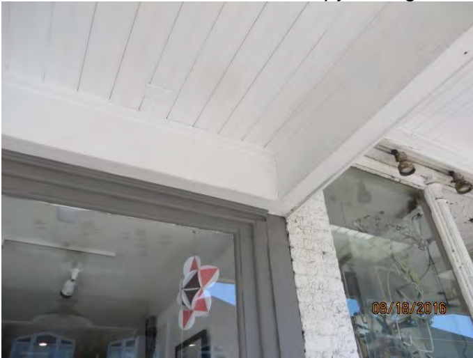
Photo 25 exterior leak from canopy ceiling
