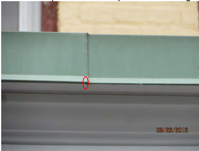
Photo 14 drip from second splice in metal edge
