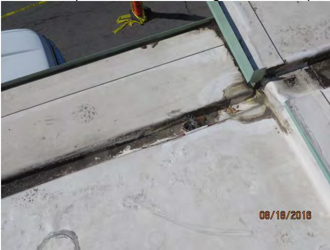
Photo 5 exposed wood blocking rotted at step between roof levels
