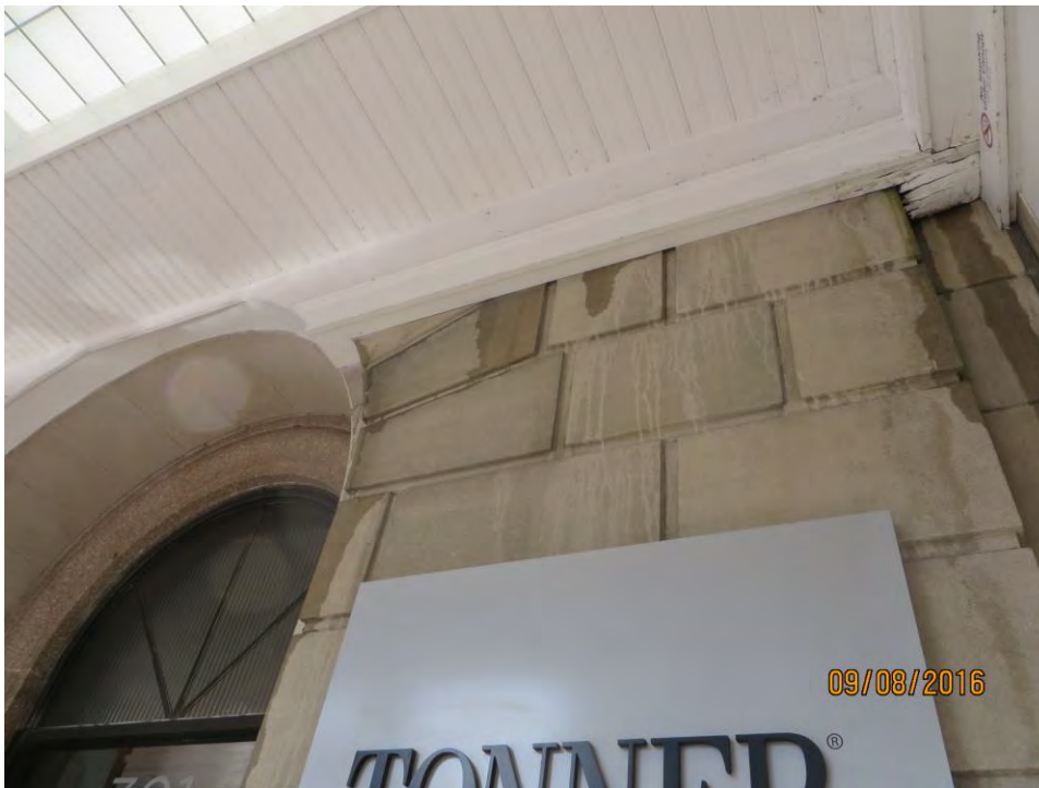
Photo 14 water running down the wall directly below the water test area at 10:23 AM.
