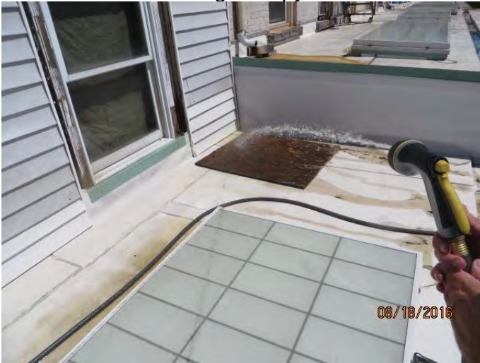
Photo 26 water testing canopy
