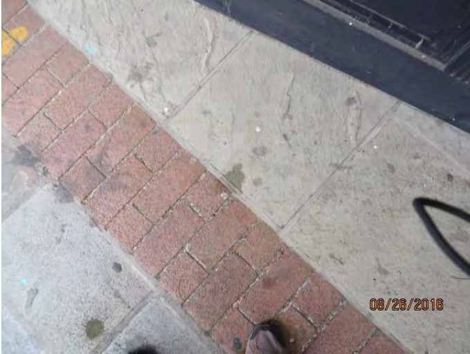
Photo 28 Drops on sidewalk second water leak at vestibule at 11:18 AM
