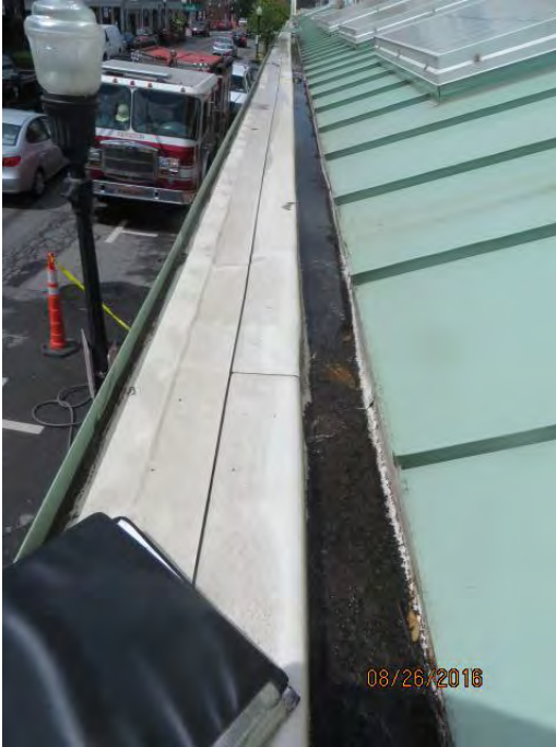
Photo 8 Partially filled gutter
