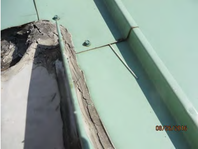
Photo 7 five inch long probe inserted between metal roof panel splice
