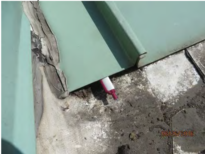
Photo 3 pen inserted between roof membrane and metal roof panel
