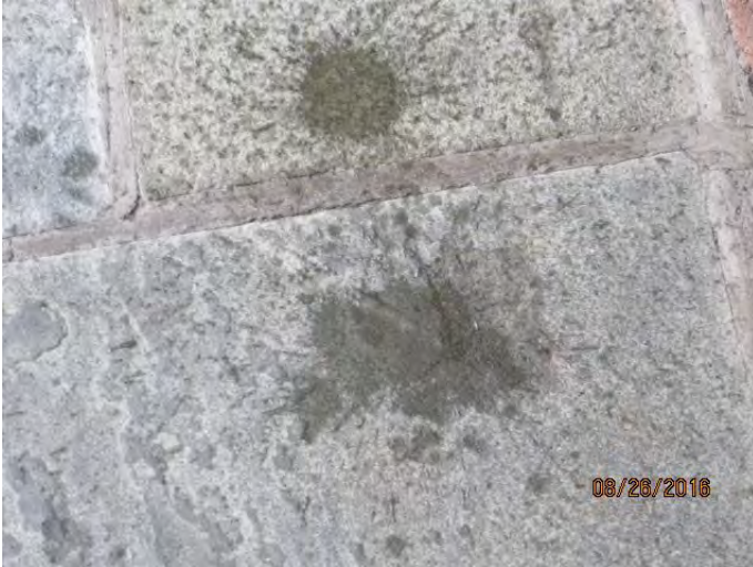
Photo 30 Drops on side walk from water leaks at North Skylight
