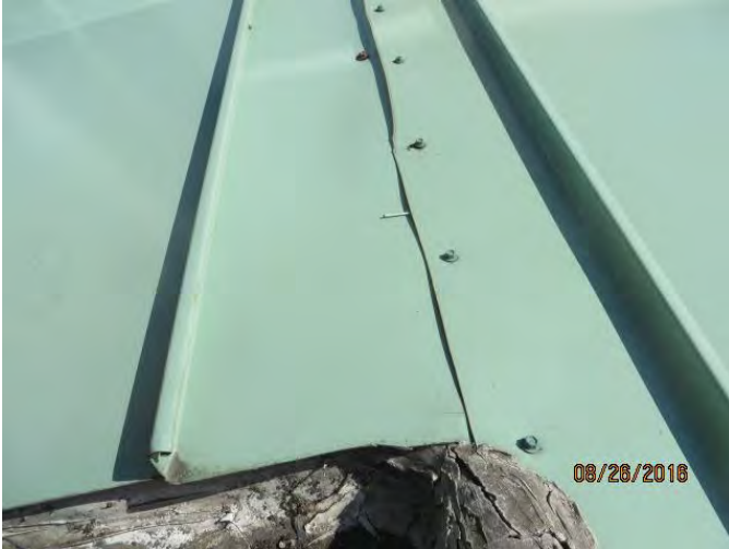
Photo 8 five inch probe inserted into metal panel side lap
