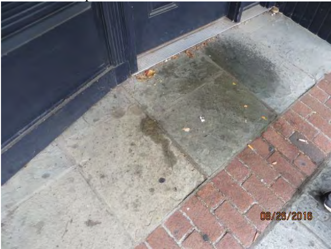
Photo 32 Drops on sidewalk from water leak at vestibule light at 11:24 AM
