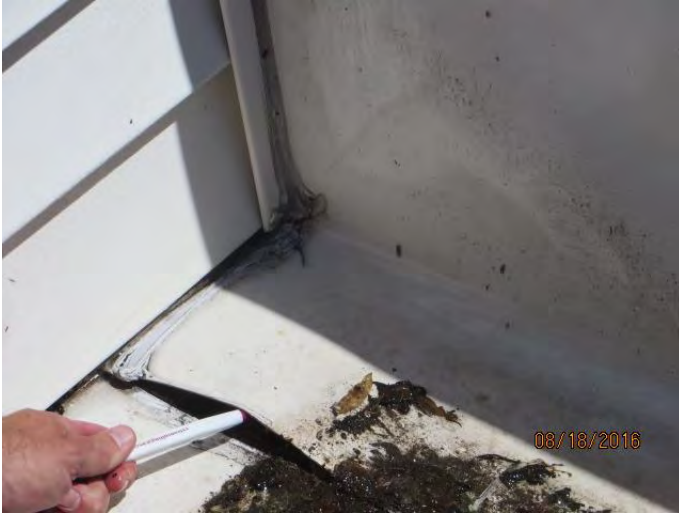
Photo 28 roof membrane opening over exterior leak location
