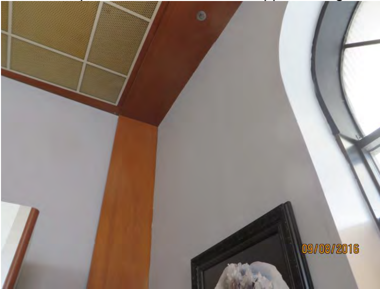
Photo 3 Reported location of leak in upper ceiling corner
