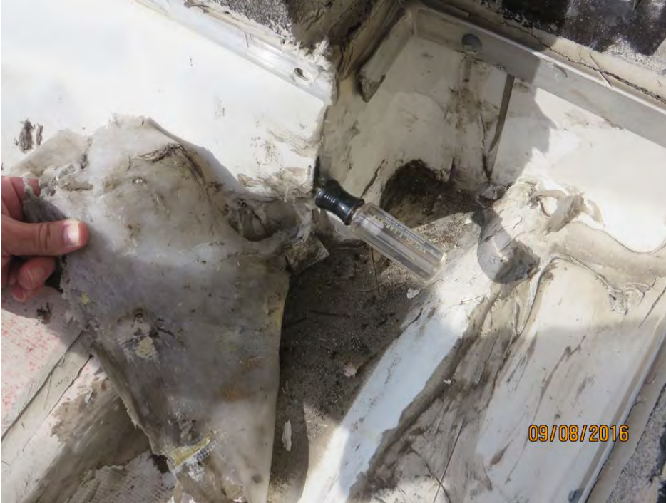
Photo 7 Flashing repair is not attached to roof membrane and seam probe inserted into flashing opening
