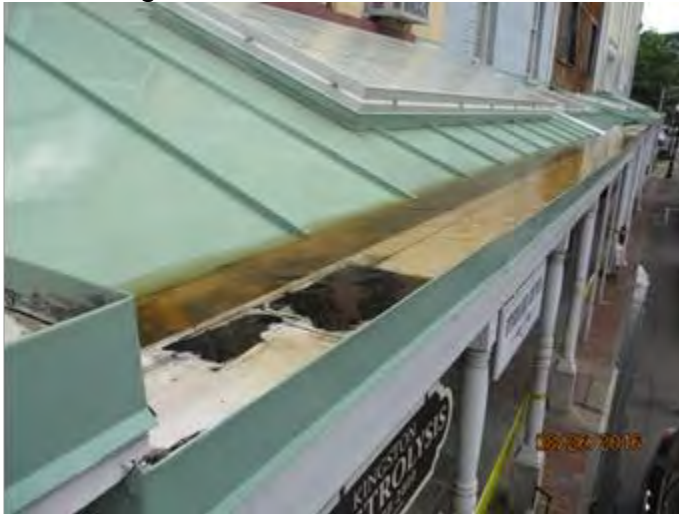
Photo 11 gutter filled with water
