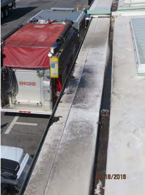
Photo 3 gutter partially plugged
