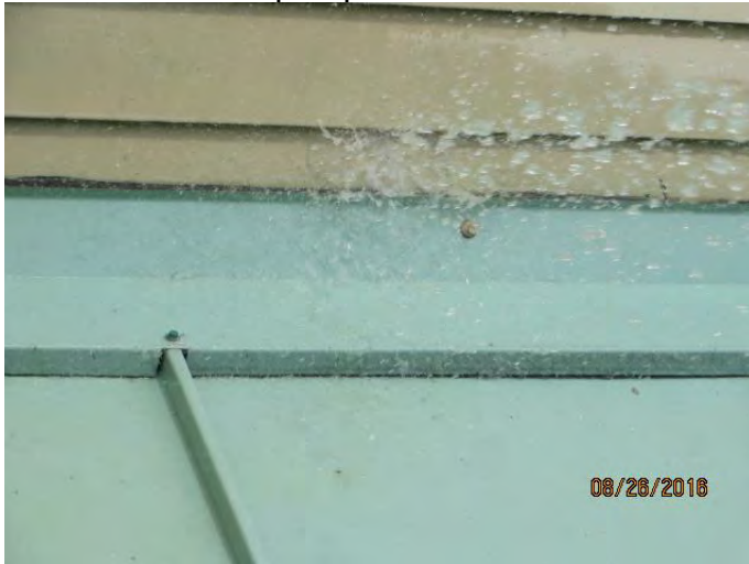
Photo 13 Close up of photo 12
