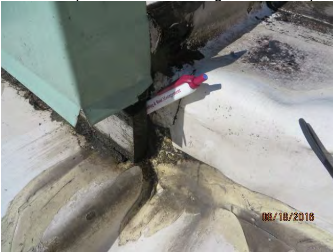
Photo 6 exposed wood blocking rotted at step between roof levels
