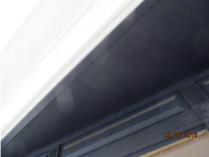
Photo 27 Second water leak at vestibule at 11:18 AM
