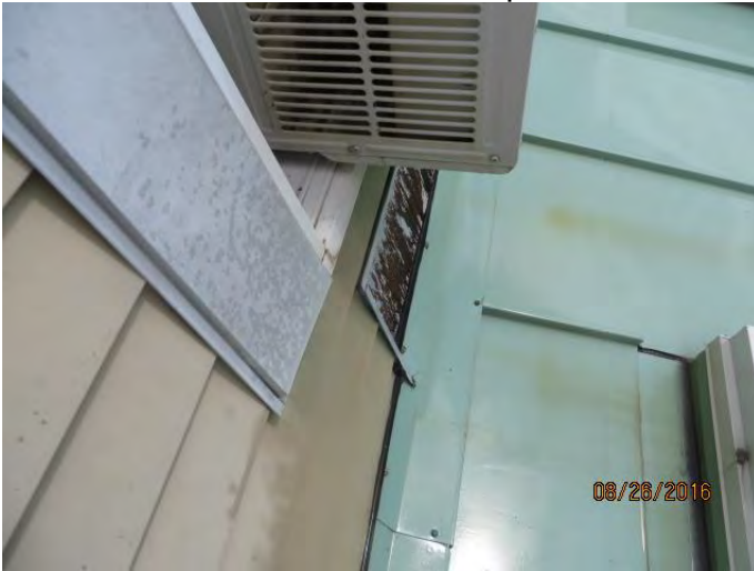
Photo 9 Deteriorated wood infill panel below air conditioner
