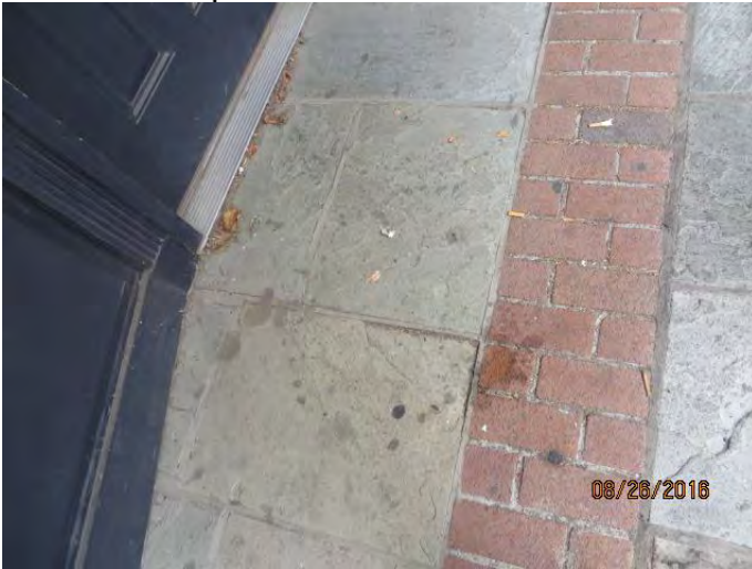
Photo 22 Drops on sidewalk from Water leak at vestibule at 11:17 AM
