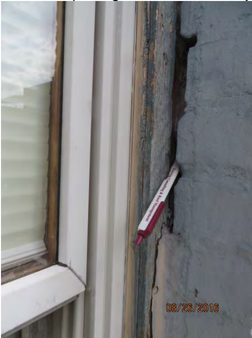
Photo 7 Opening between window jamb frame and brick wall, see pen in opening
