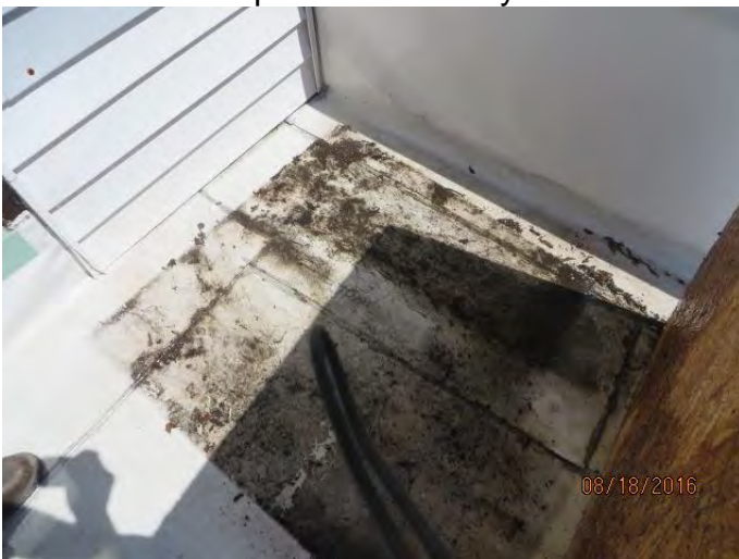
Photo 27 lifted up wood in vicinity of exterior leak
