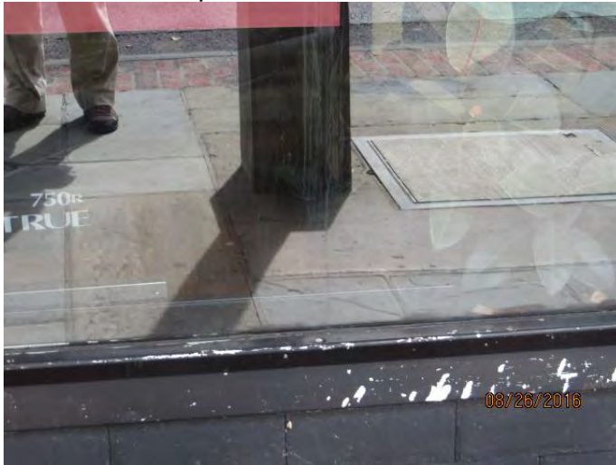
Photo 4 Below photo 2, see dried water streaks and peeled paint
