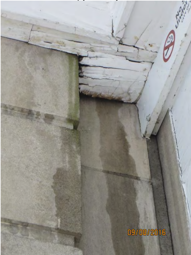
Photo 10 At 10:17 AM, water observed at water stained and damaged wood on underside of canopy directly below water test
