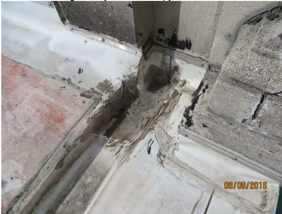
Photo 6 Flashing directly above canopy water stains and deteriorated wood
