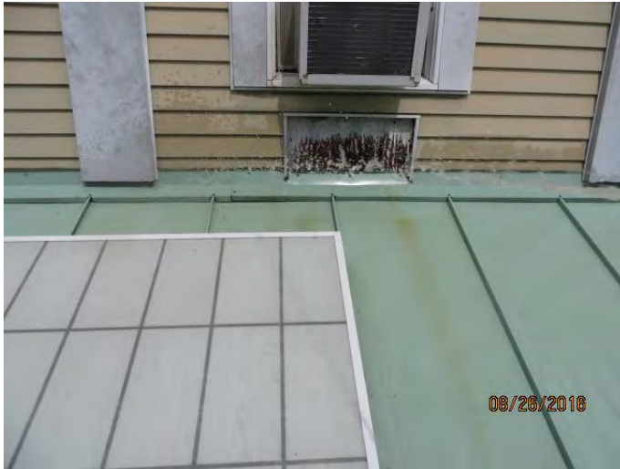
Photo 12 Water test between vertical white siding began at 12:10 PM
