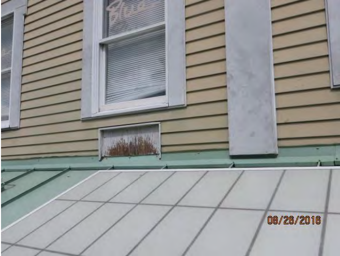
Photo 7 Deteriorated wood infill panel
