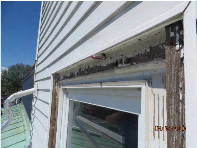
Photo 15 hole in window frame
