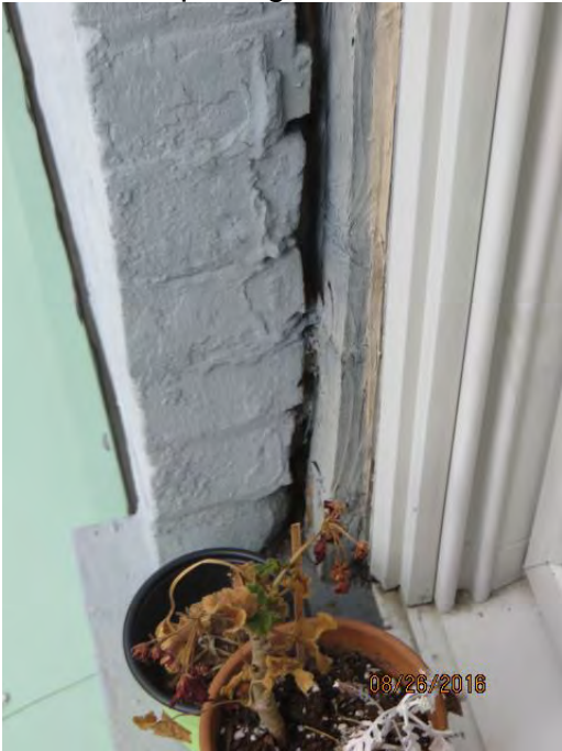
Photo 15 Opening between window jamb frame and brick wall
