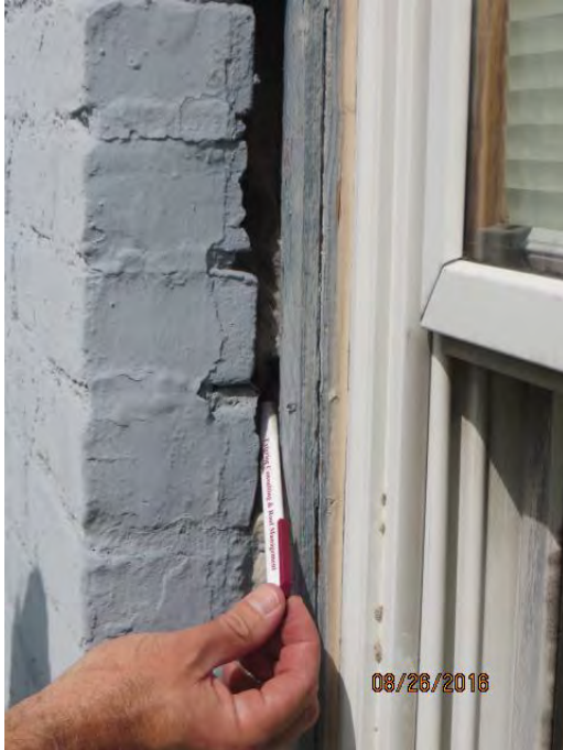
Photo 5 Opening between window jamb frame and brick wall, see pen in opening
