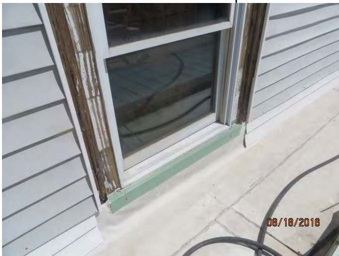
Photo 6 window above area of reported leaks
