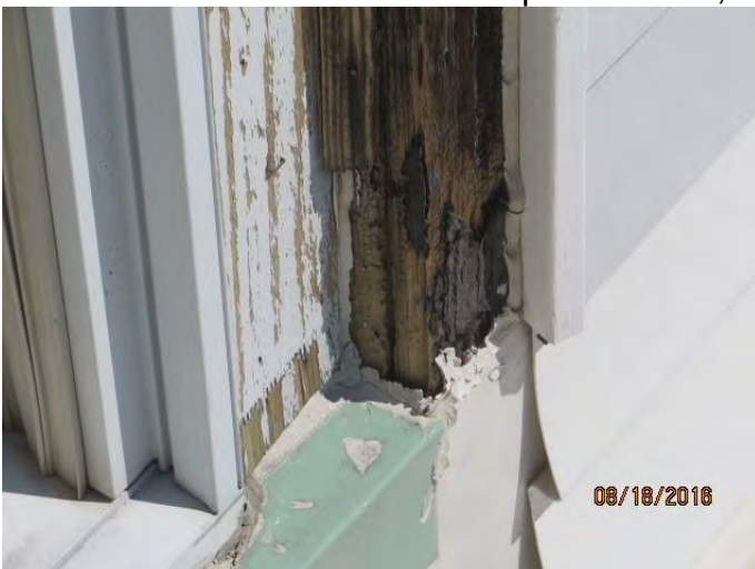
Photo 9 window above area of reported leaks, cracks in window frame
