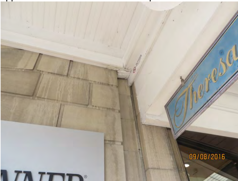
Photo 4 Water stains and deteriorated wood on the canopy underside on the opposite side of the wall from the reported leak location
