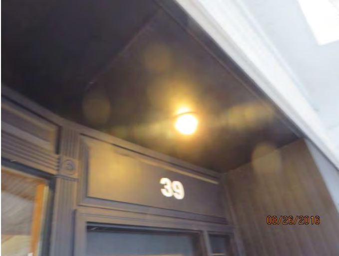
Photo 31 Water leak at vestibule light at 11:24 AM
