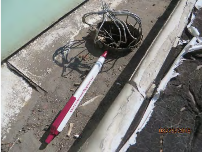
Photo 5 downspout starter lip raised above gutter botom
