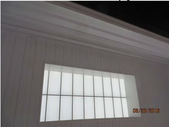
Photo 29 Water leaks at North Skylight
