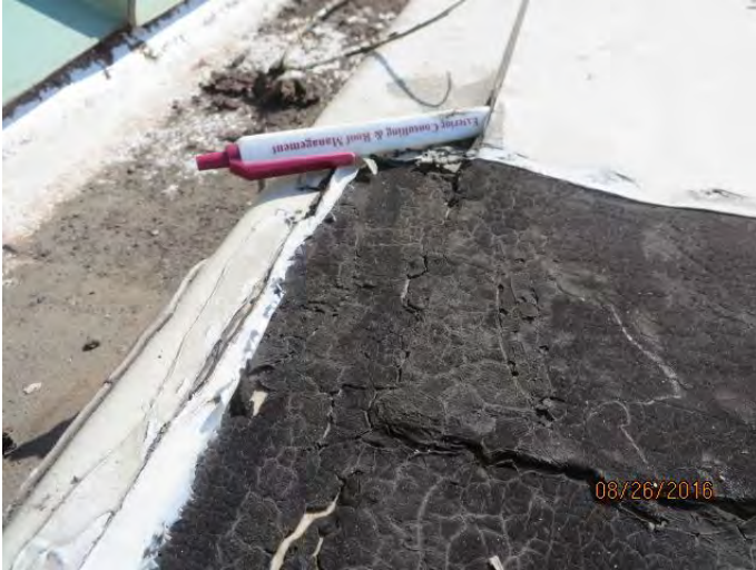
Photo 4 pen inserted into roof membrane opening at metal edge flashing
