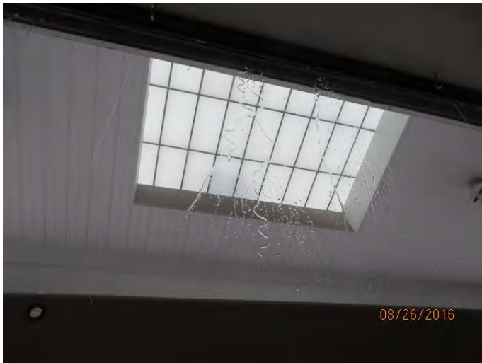
Photo 18 Water leak observed on the interior of front display window at 12:18 PM
