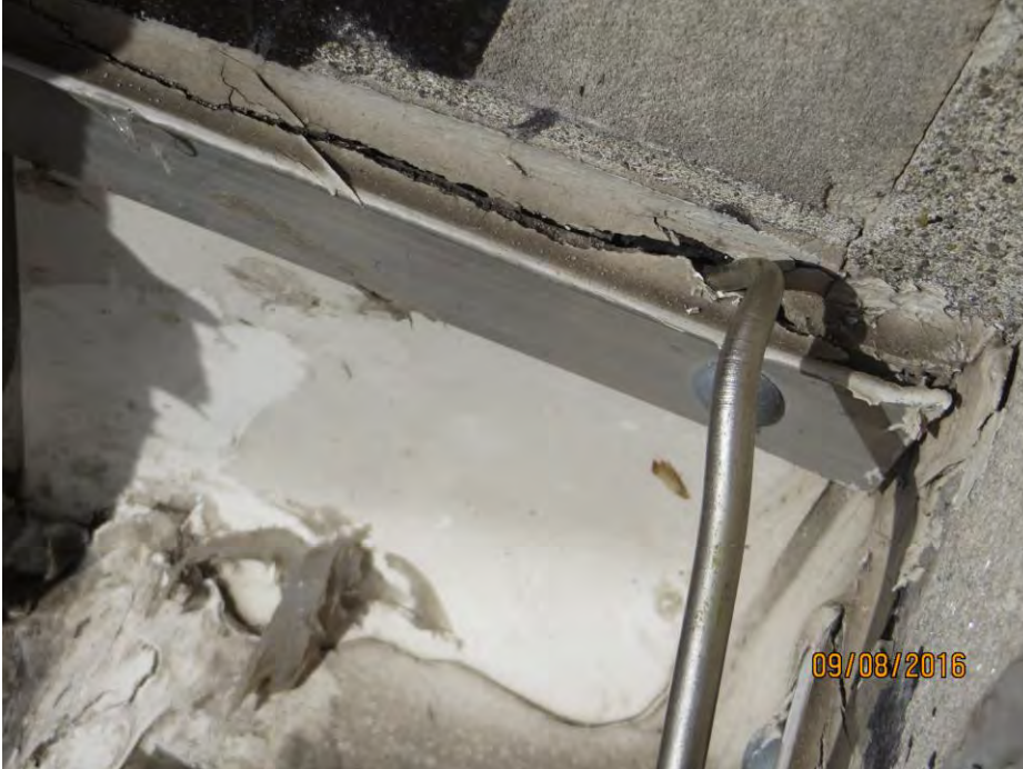
Photo 8 Crack in sealant at top of termination bar, seam probe inserted into crack
