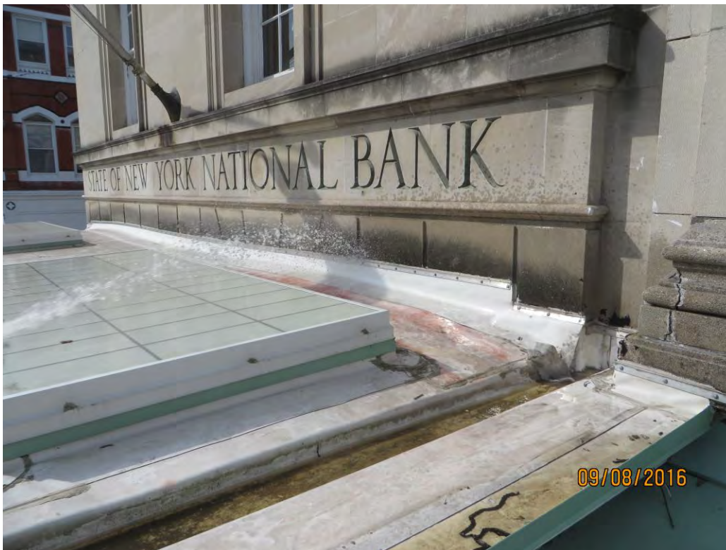
Photo 12 Commence water test at top of base flashing along the wall directly above the water stains on the wall at 10:21 AM.
