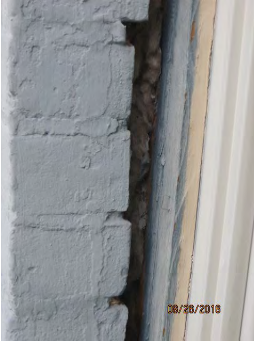
Photo 16 Opening between window jamb frame and brick wall
