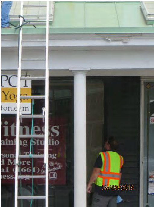
Photo 17 General location of leak in photo 14
