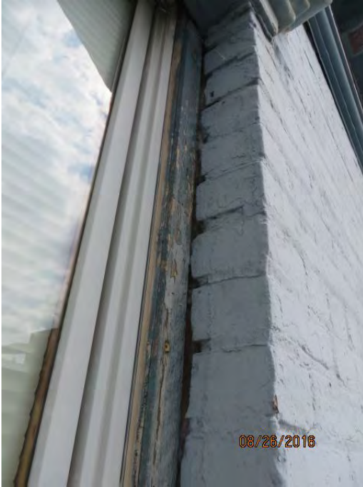
Photo 8 Opening between window jamb frame and brick
