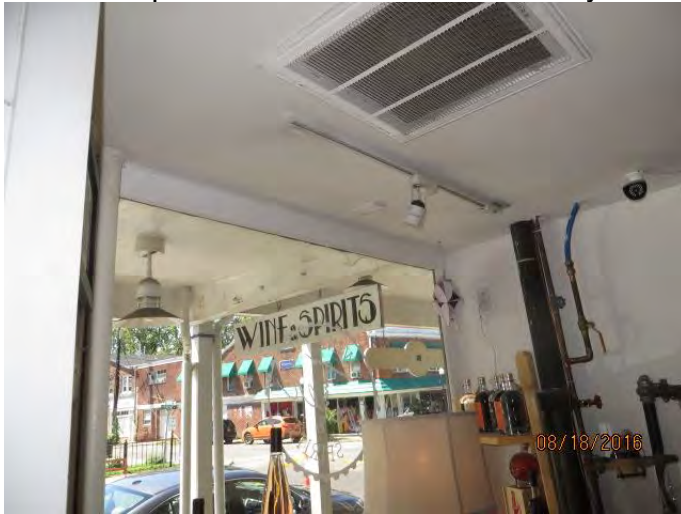
Photo 5 reported area of leaks after heavy blowing rain
