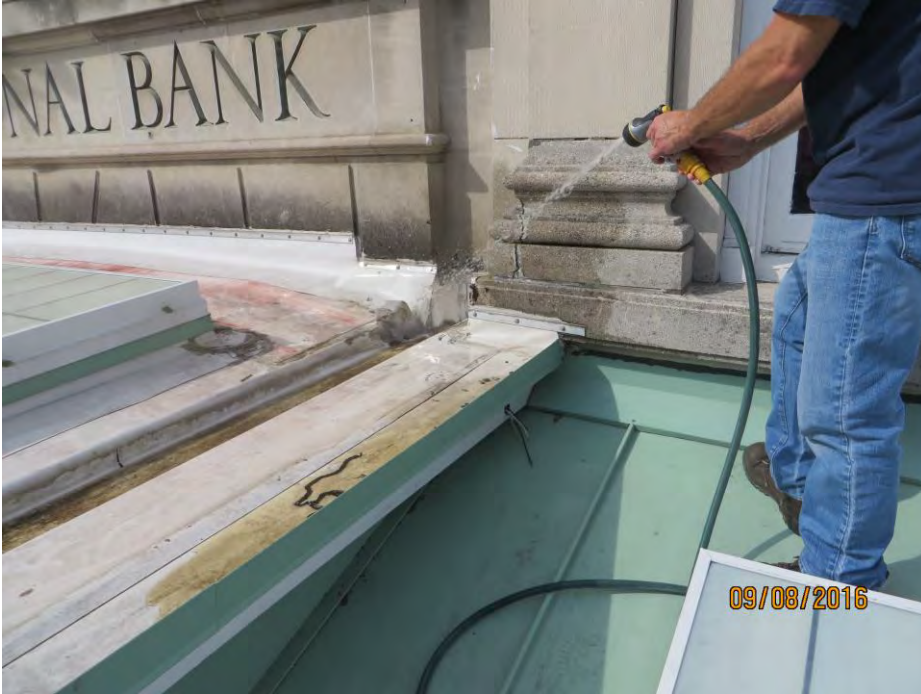
Photo 9 Commence water test at 10:16 AM
