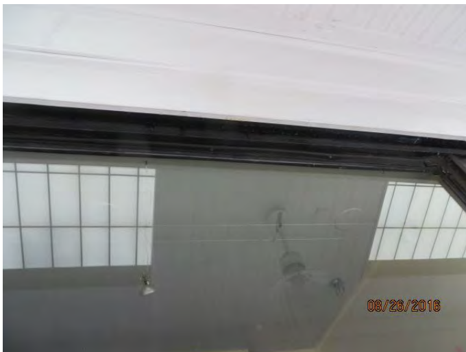
Photo 14 Water leak observed at upper exterior of front display window at 12:12 PM
