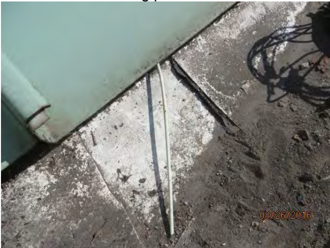
Photo 6 five inch long probe inserted between roof membrane and metal panel
