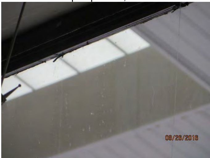
Photo 3 Close up of photo 2, see dried water streaks
