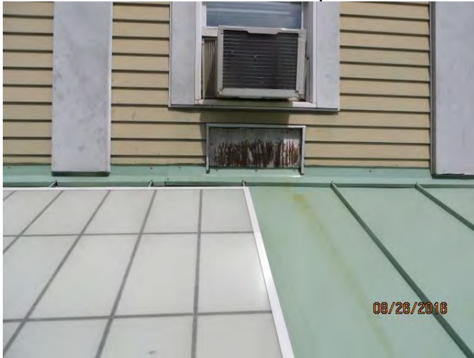
Photo 5 Deteriorated wood infill panel below air conditioner
