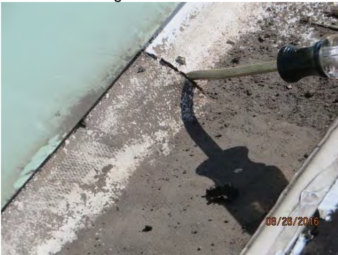
Photo 9 Void in gutter roof membrane
