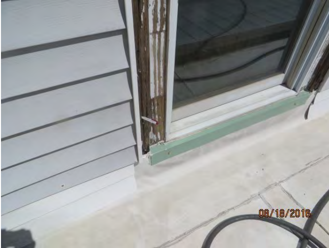
Photo 7 window above area of reported leaks, see pen in window frame opening
