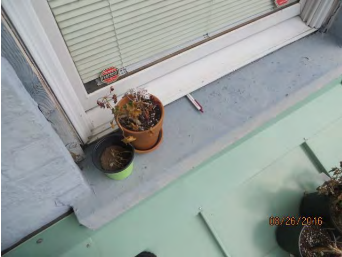
Photo 10 Opening between window sill frame and stone sill, see pen in opening
