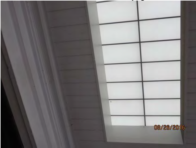
Photo 24 Water leak at south skylight at 11:17 AM
