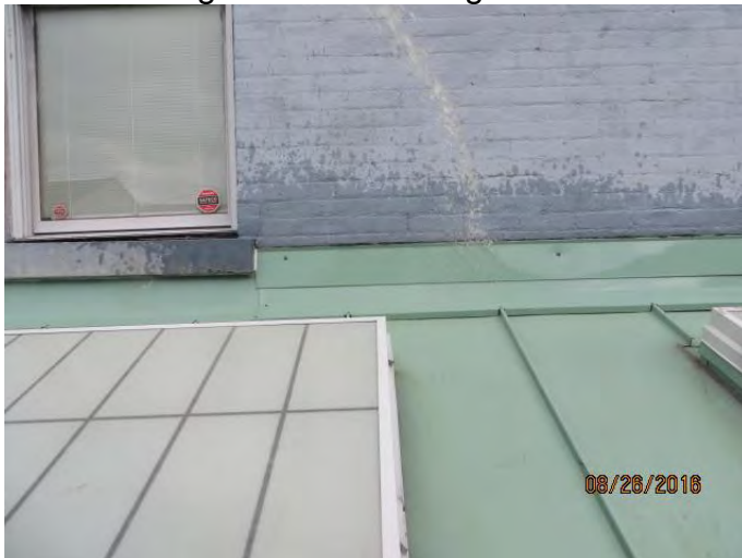
Photo 20 Began water test of green metal base flashing at 11:14 AM
