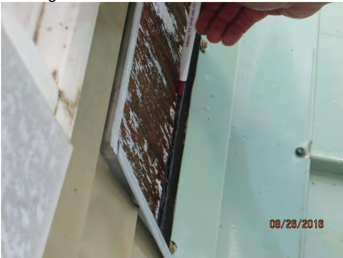
Photo 10 Opening between deteriorated wood infill panel and green metal base flashing
