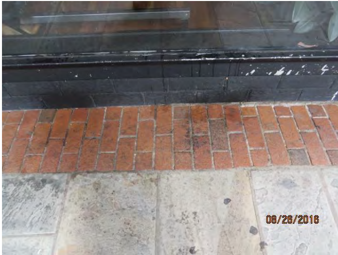
Photo 16 Water on side walk beneath leak shown in photo 14 and 15
