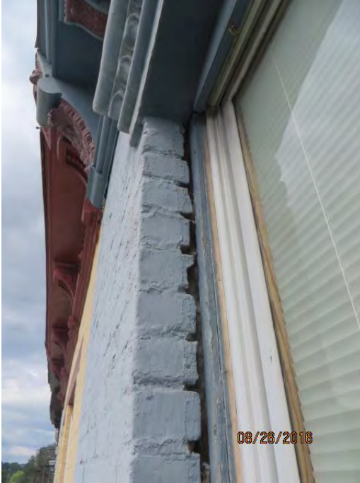
Photo 6 Opening between window jamb frame and brick
