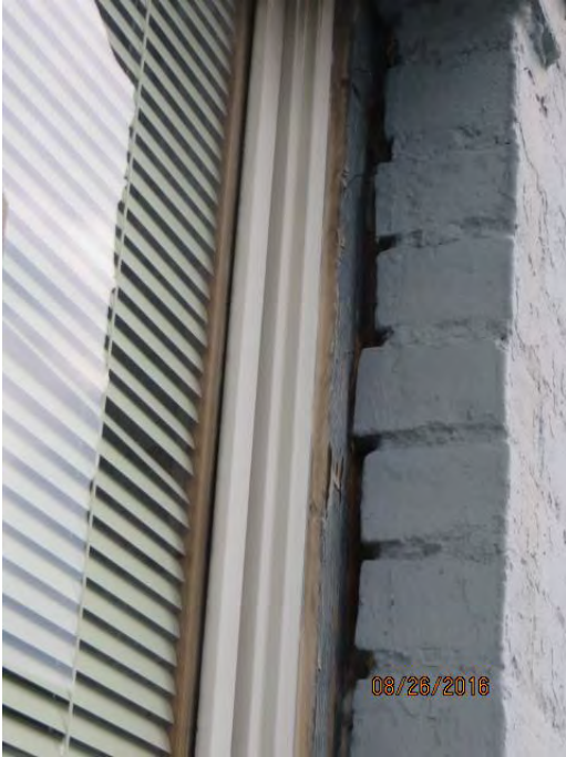
Photo 14 Opening between window jamb frame and brick wall
