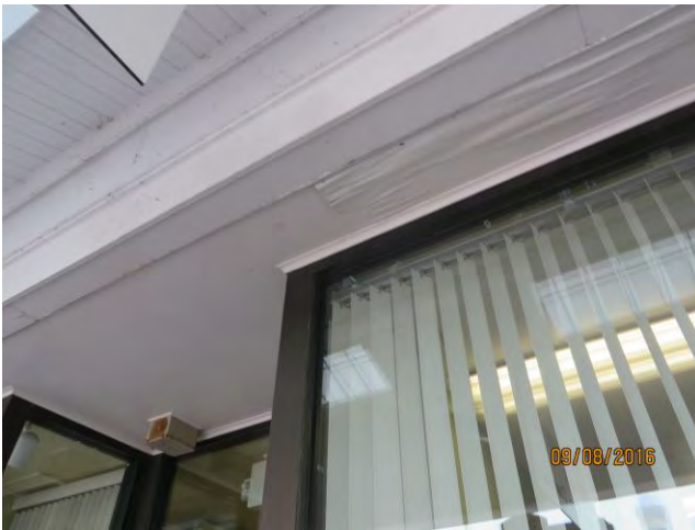
Photo 13 At 10:48 AM, water drops appeared on the soffit below the water test area
