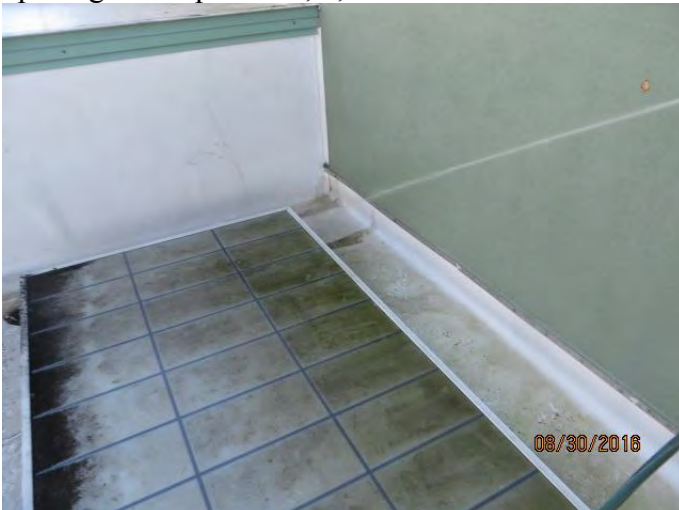
Photo 33 Start water test at west end of 44 N. Front St. at 9:51 AM at roof membrane openings from photos 4, 5, 6 and 7.
