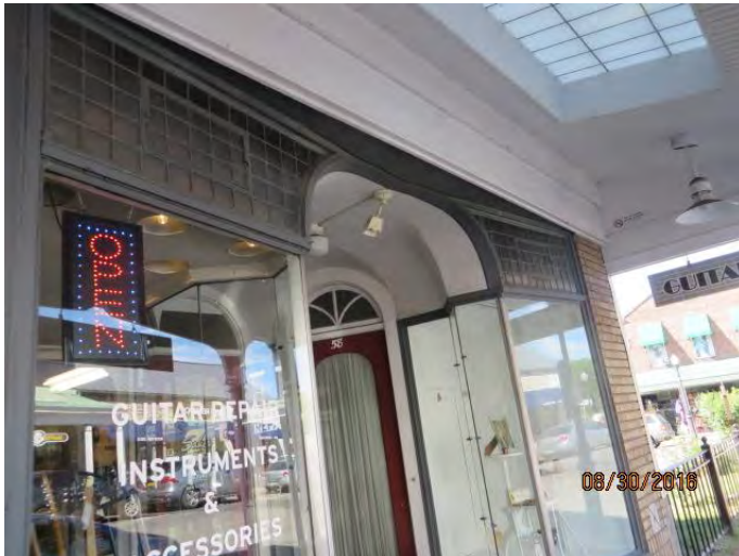
Photo 9 Water leaks observed across the front of 58 N. Front St. at 11:09 AM
