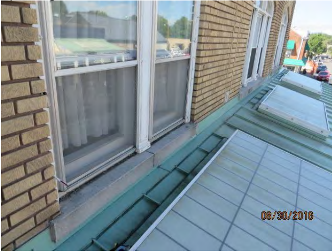
Photo 6 Roof canopy over 54 North Front Street, see pen in large window jamb opening
