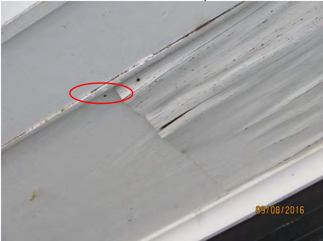
Photo 14 soffit with water drops. The water drops are difficult to see in the photo
