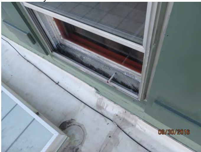
Photo 23 Eighth window from the west end, outer closure not closed, allows water entry
