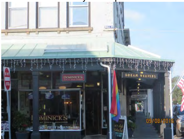
Photo 16 Previously not reported leak at top of column near white downspout
