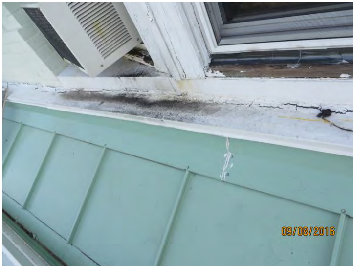
Photo 11 Water table crack continues across the building's front
