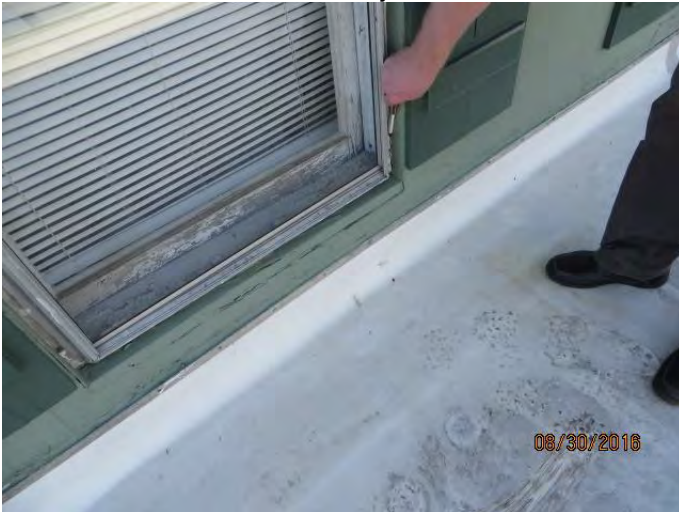
Photo 13 Crack in window jamb sealant
