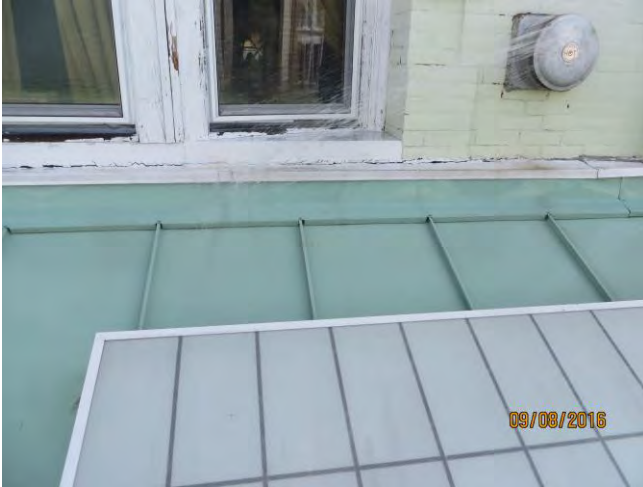
Photo 12 Begin water test at 10:47 AM across the building's front focusing on the water table crack with window sills taped
