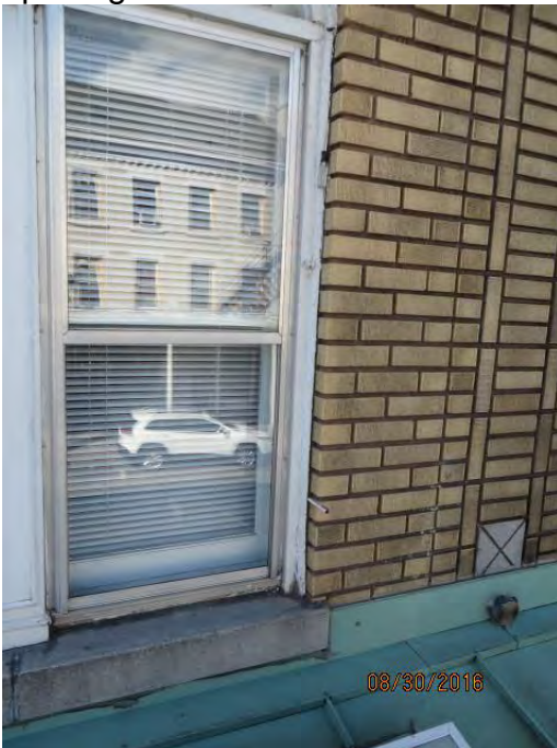
Photo 5 Roof canopy over 54 North Front Street, see probe in large window jamb opening
