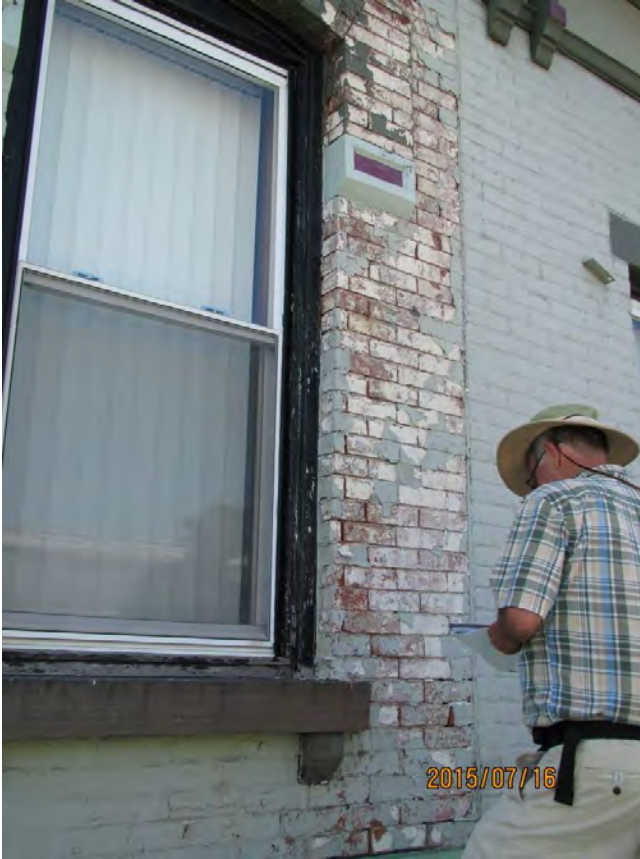
Photo 10 brick wall mortar joints above the canopy are deteriorated
