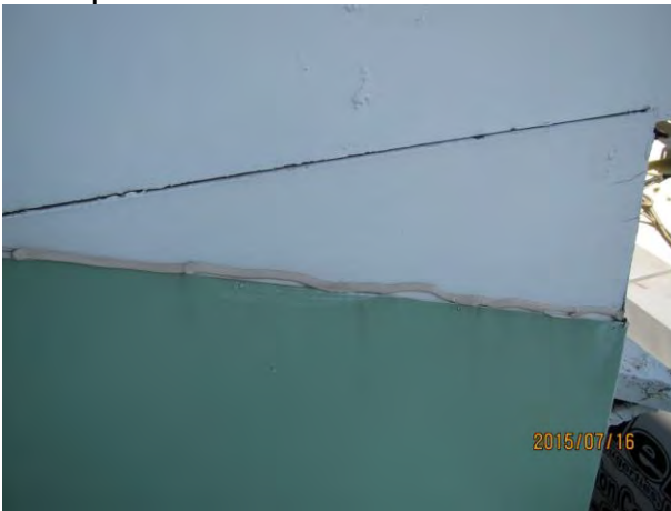
Photo 13 metal base flashing is open at the top and no metal counter flashing at the top
