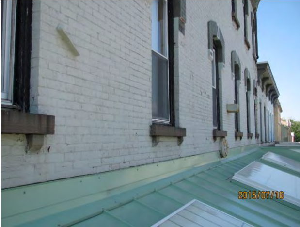
Photo 4 Leaks reported inside the building beneath the top of the green metal roof where it contacts the building
