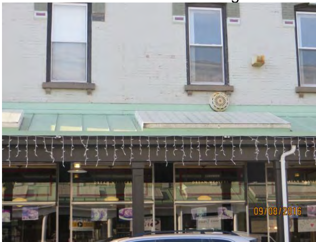
Photo 3 Leaks reported inside the building beneath the top of the green metal roof where it contacts the building
