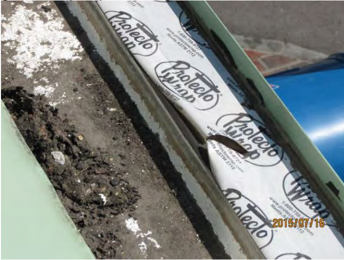
Photo 18 Improper flashing material (Protecto Wrap) used to flash metal edge gravel stop adjacent to gutter
