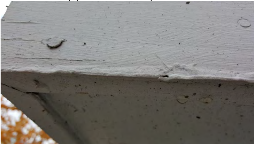
Photo 6 Close up photo 5, water drips are difficult to see
