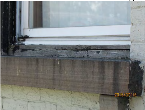
Photo 9 wood window sills above canopy are deteriorated
