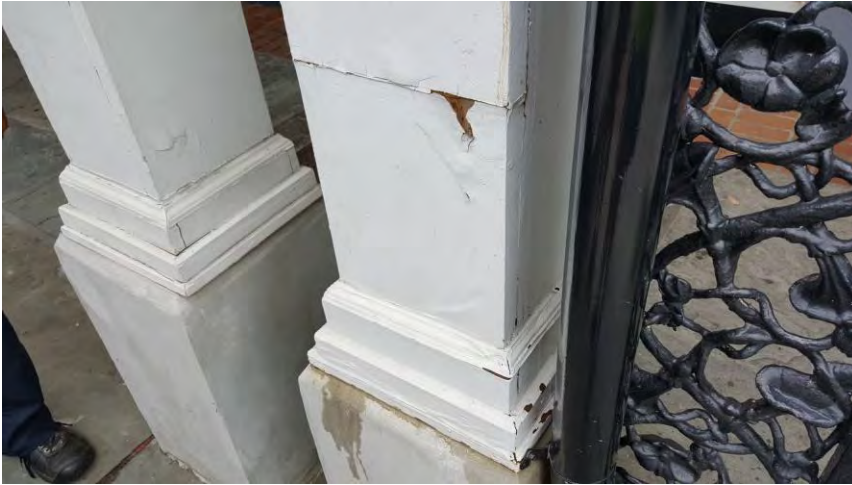
Photo 4 Previously unreported water damage to column between 38 and 40 North Front St
