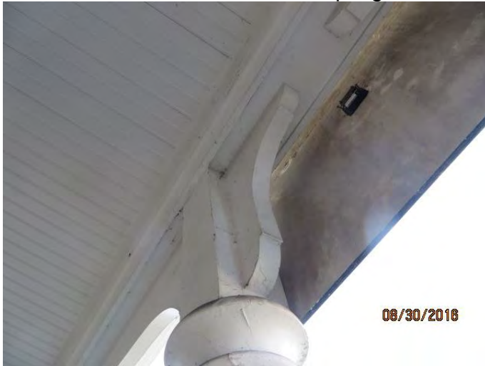
Photo 16 Leak behind Clock Shop sign
