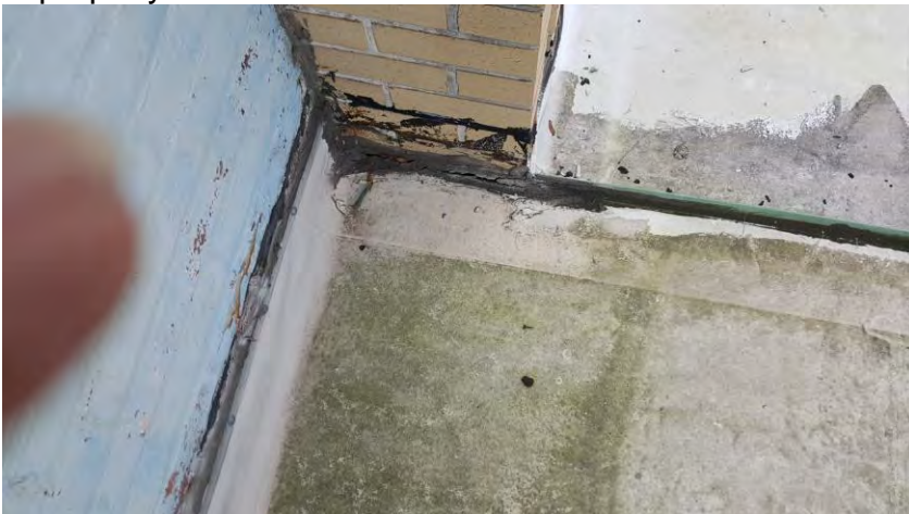
Photo 3 Directly above the water stained ceiling tile, the roof was found to be improperly terminated to the brick wall.
