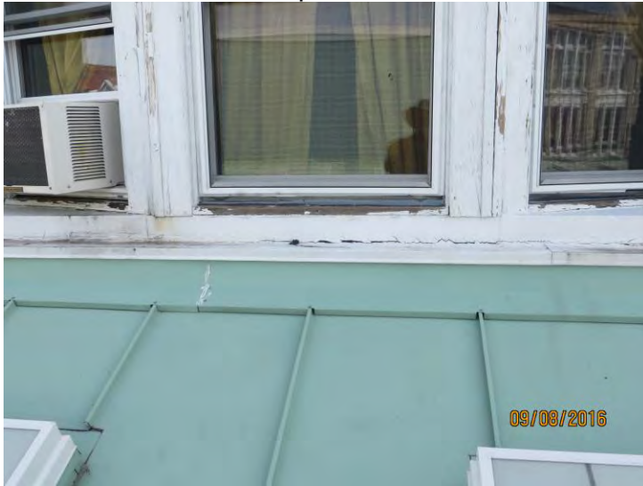
Photo 7 Window sills taped off for water test
