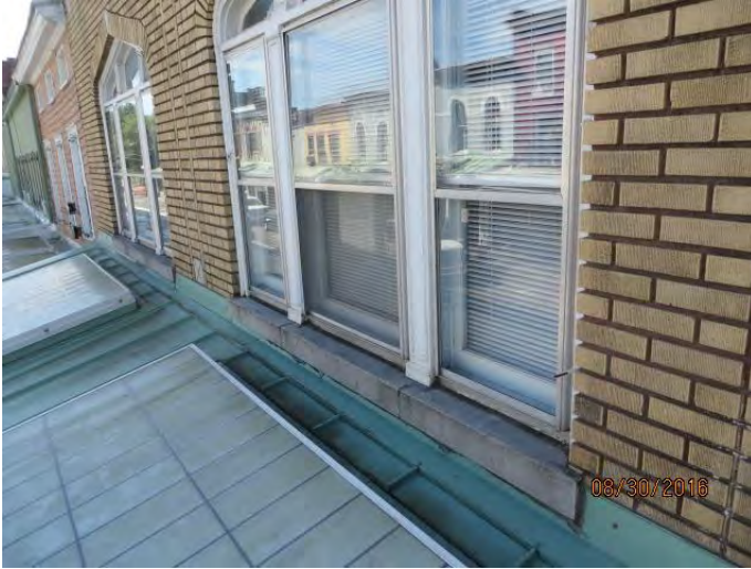
Photo 4 Roof canopy over 54 North Front Street
