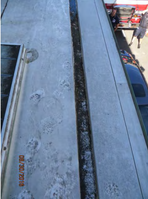
Photo 2 gutter partially filled
