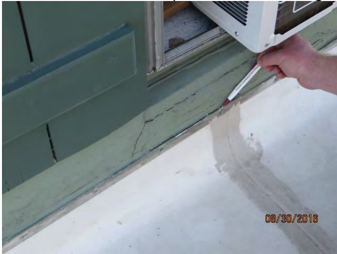
Photo 19 Crack at the top of the base flashing
