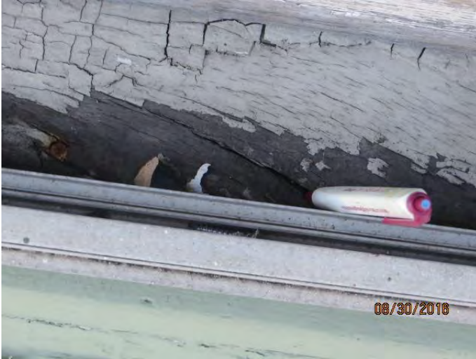
Photo 25 Eighth window from west end, crack in window sill frame
