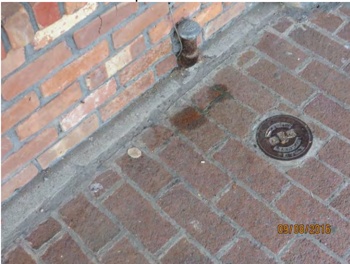
Photo 17 water drops on sidewalk beneath soffit of photo 16
