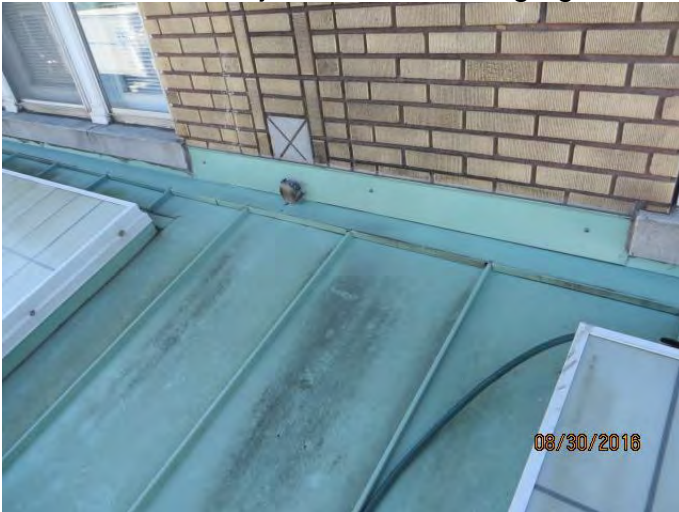
Photo 9 Electrical junction box through green metal base flashing
