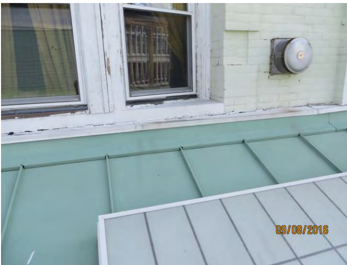
Photo 5 Window sills above metal canopy has large openings that were taped off for the water tests
