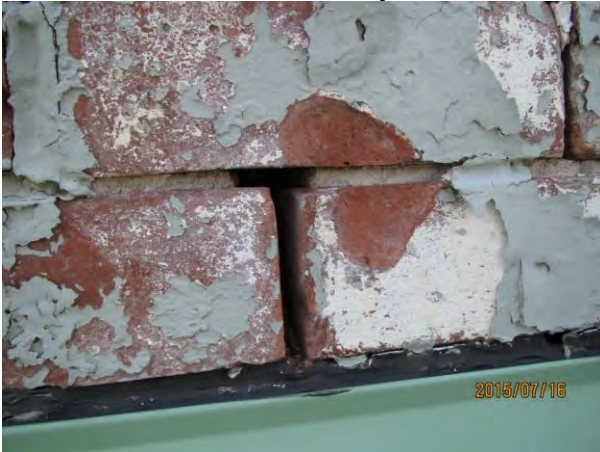
Photo 12 brick wall mortar joints above the canopy are deteriorated
