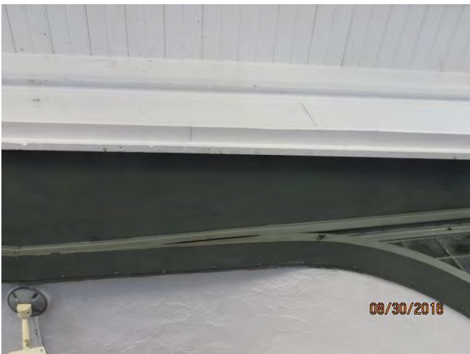
Photo 21 Second Water leak at fascia of front entrance
