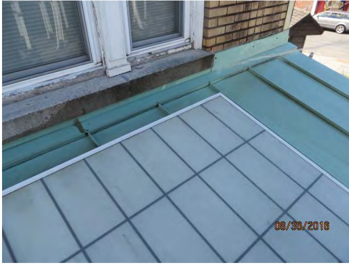
Photo 7 Begin water test on green metal base flashing at 11:08 AM across width of 58 N. Front St.
