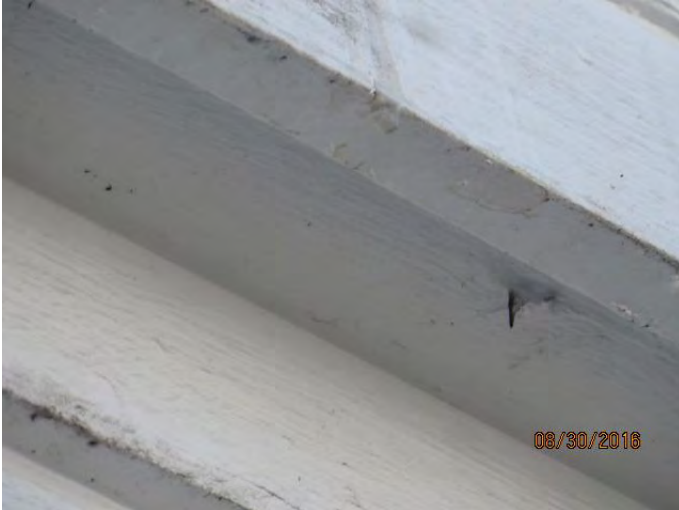
Photo 14 Close up of photo 13, see water drops
