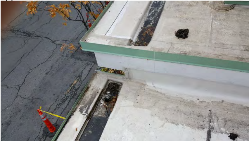
Photo 5 Above damaged column, gutter is plugged and water dripping down from upper fascia
