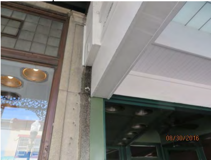
Photo 35 At 9:52, leaks observed between 42 and 44 North Front St directly beneath water test of photos 33 and 34
