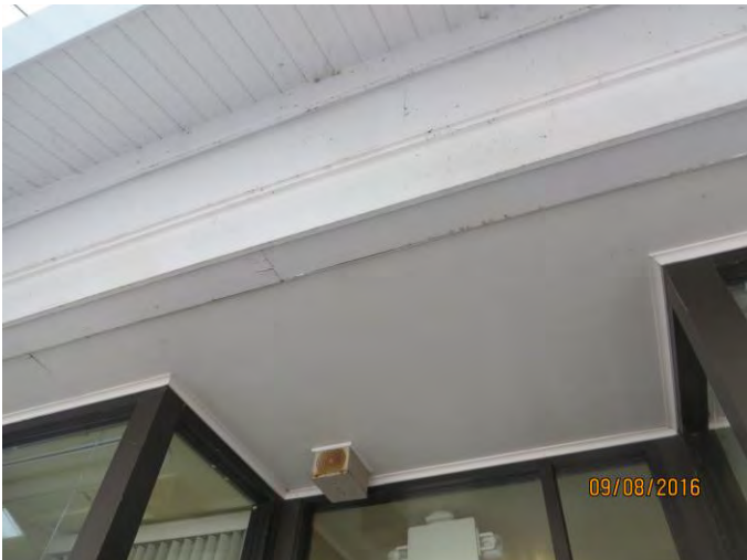
Photo 3 Water stains on soffit
