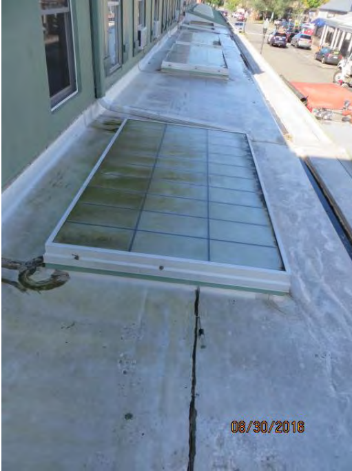
Photo 8 Opening in roof membrane west side of near skylight
