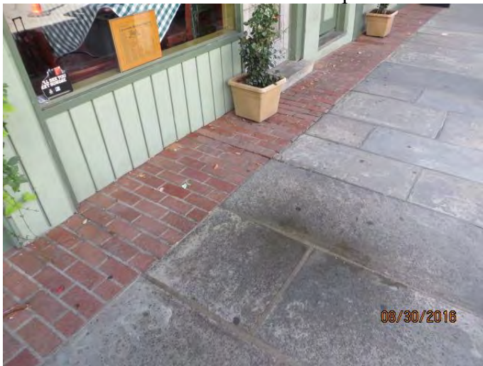
Photo 41 Water on sidewalk beneath photo 40
