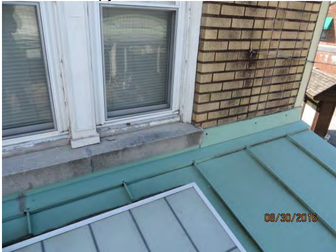
Photo 2 Canopy roof over 58 N. Front St.
