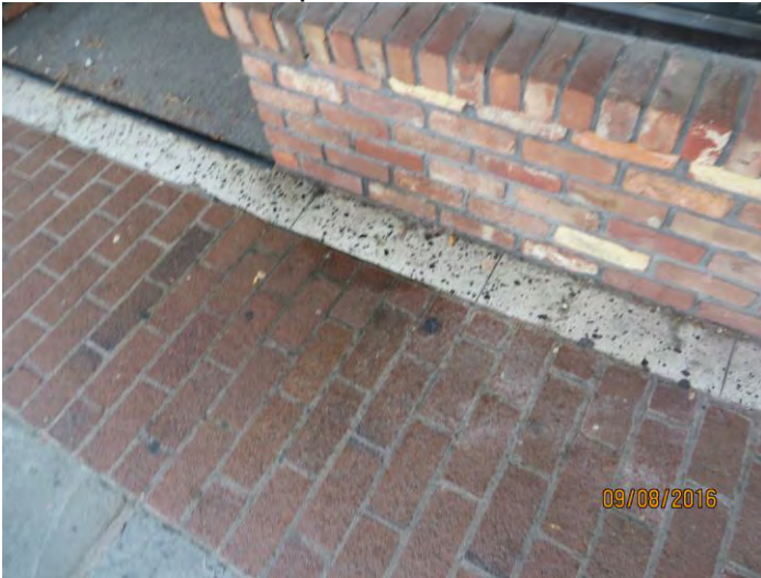
Photo 15 water drops on side walk below soffit
