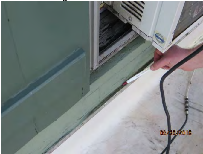
Photo 29 Ninth window from the west end (farthest east), cracks in sealant at top of base flashing
