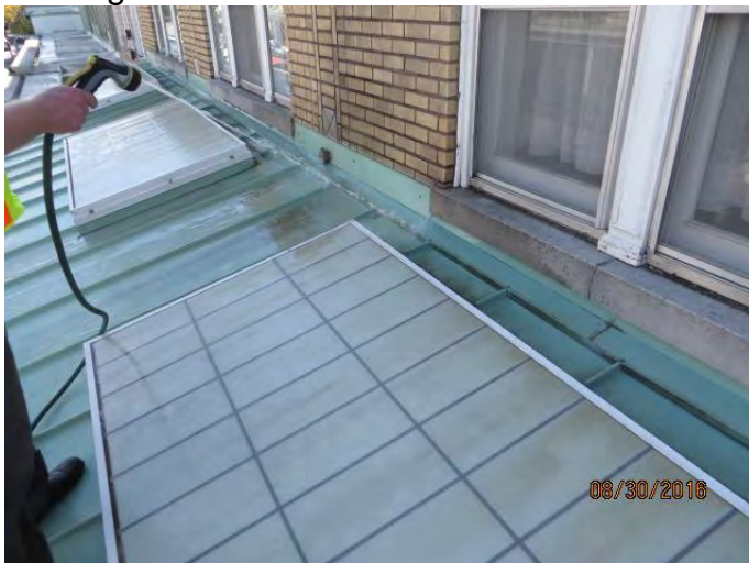
Photo 12 continuing water test at green metal base flashing across width of building
