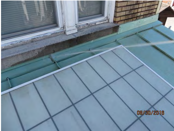
Photo 8 Begin water test on green metal base flashing at 11:08 AM across width of 58 N. Front St.
