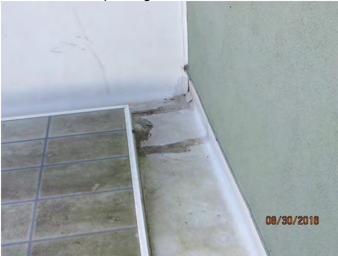
Photo 4 Two openings in roof membrane
