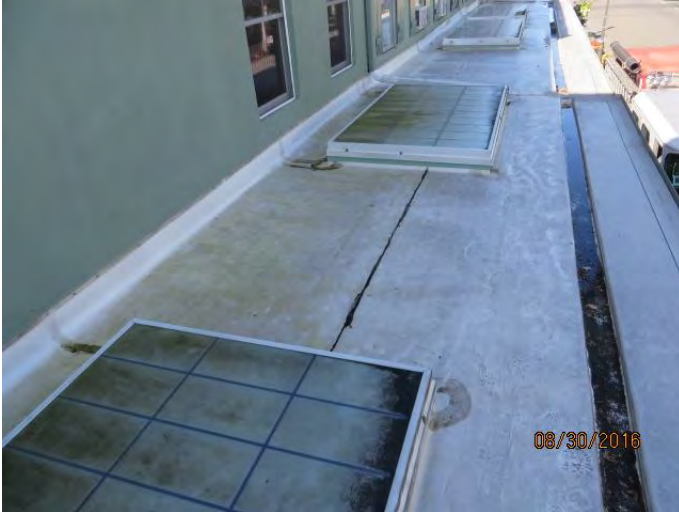
Photo 1 Canopy roof over 44 North Front St at west end looking east.
