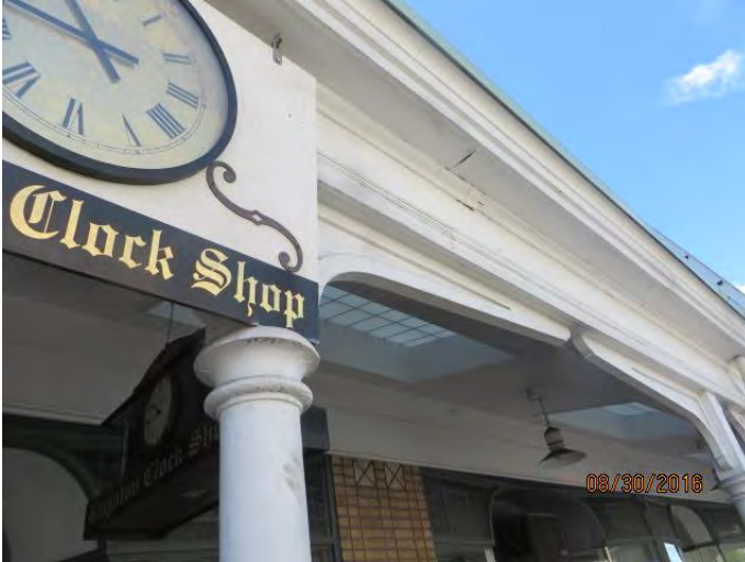
Photo 13 Water leak observed at fascia not previously reported
