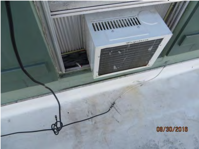
Photo 27 Ninth window from the west end (farthest east), air conditioner closure not at window exterior, allows water entry
