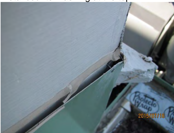
Photo 14 top view of photo 13, metal base flashing is open at the top and no metal counter flashing at the top
