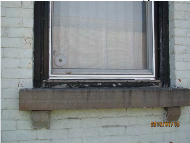
Photo 9 wood window sills above canopy are deteriorated
