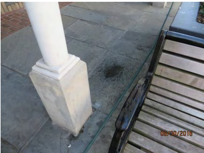
Photo 15 Water on side walk beneath fascia leak
