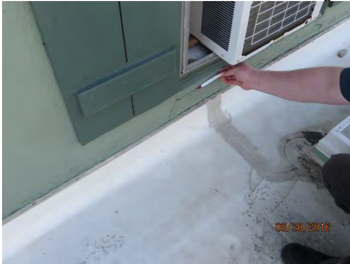
Photo 17 Crack in wood above base flashing
