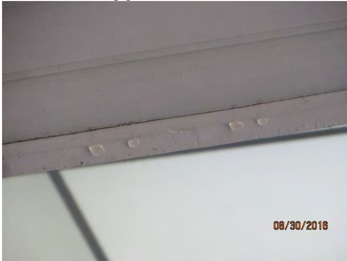
Photo 40 Close up photo 39
