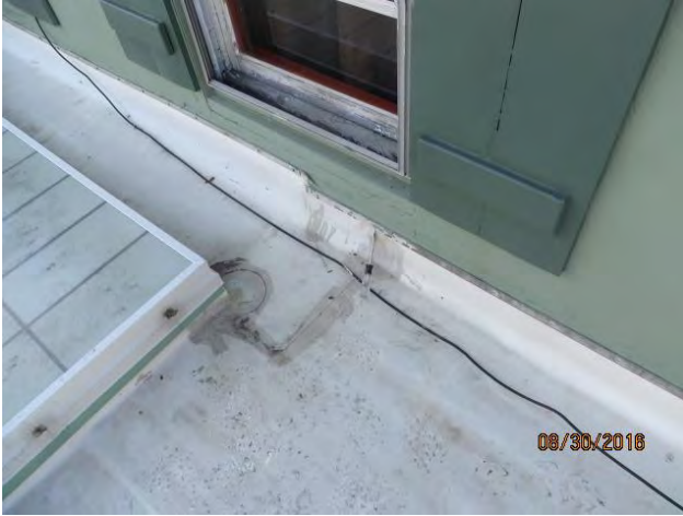
Photo 31 Eighth window from west end, opening in base flashing
