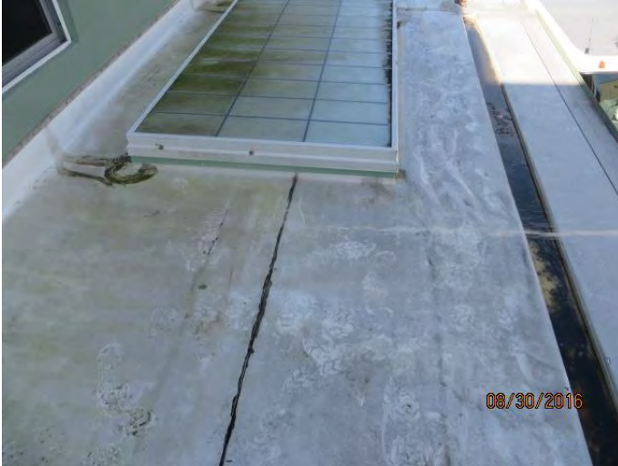
Photo 37 Water test on roof membrane opening of photo 8 and 9 at 9:56 AM
