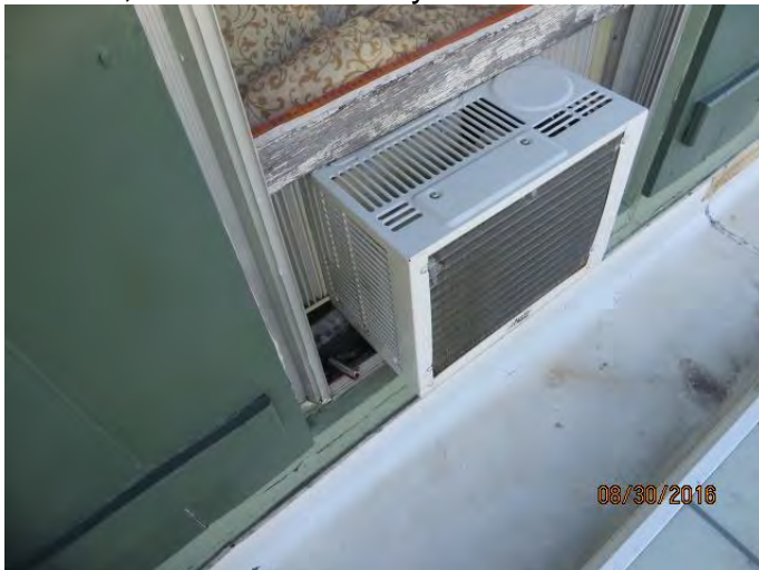
Photo 21 Sixth window from the west end, air conditioner closure not at window exterior, allows water entry
