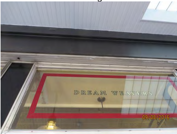
Photo 6 leaks reported along the window line beneath where the green metal roof contacts the building
