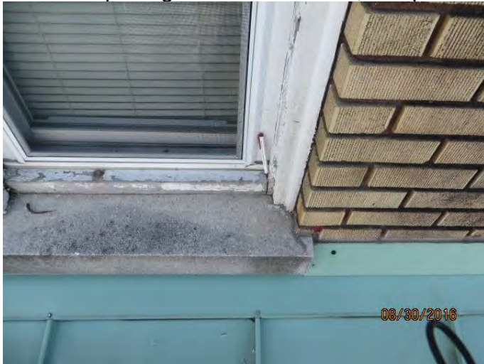
Photo 5 Opening in window sill trim, see pen
