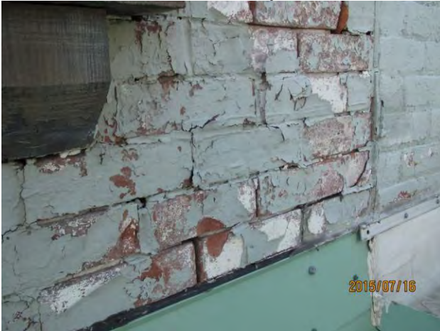
Photo 11 brick wall mortar joints above the canopy are deteriorated
