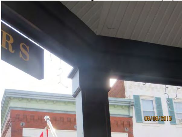
Photo 15 leaks through the column top, previously not reported
