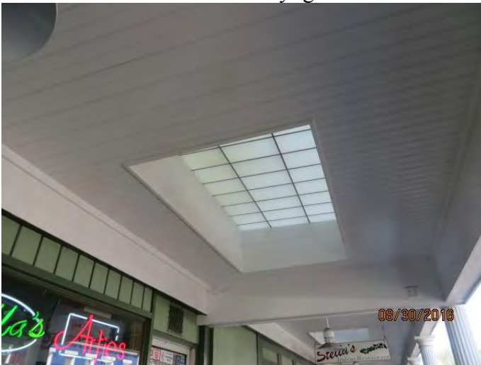
Photo 38 Water observed at skylight fascia at 10:05 AM beneath water test of photo 37
