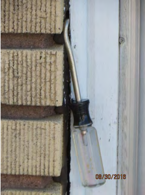
Photo 8 Probe in large window jamb opening
