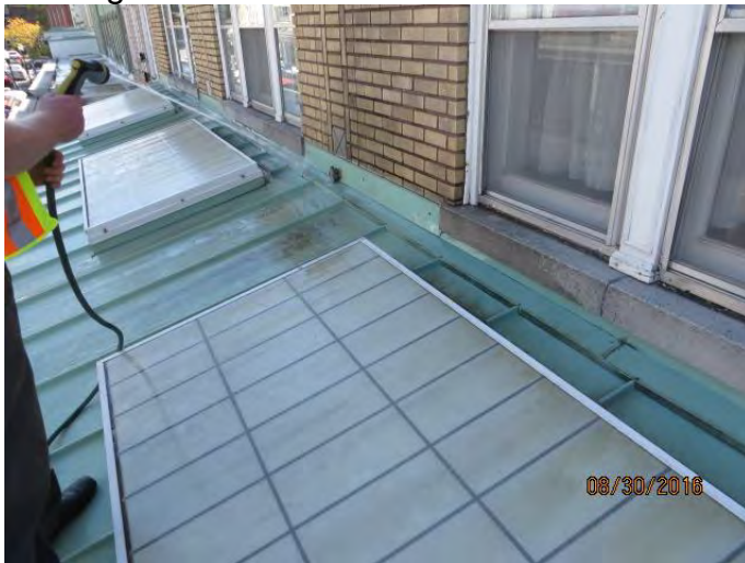
Photo 11 Begin water test at green metal base flashings across the width of building
