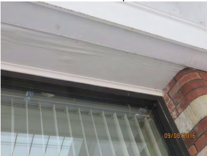
Photo 16 additional water drops at soffit
