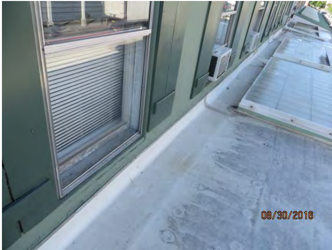
Photo 10 Crack in wood below window
