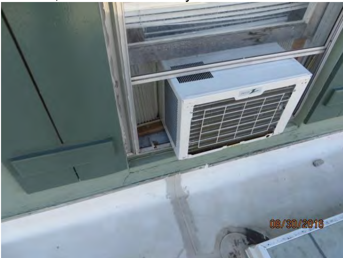
Photo 15 Fifth window from the west end, air conditioner closure not at window exterior, allows water entry
