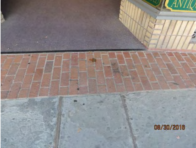
Photo 20 Water on sidewalk beneath leak shown in photo 19
