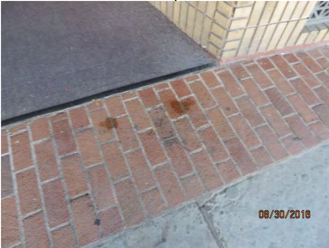
Photo 23 Second water spot on sidewalk beneath leak shown in photo 21
