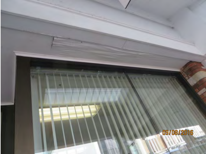
Photo 2 Water damage to soffit
