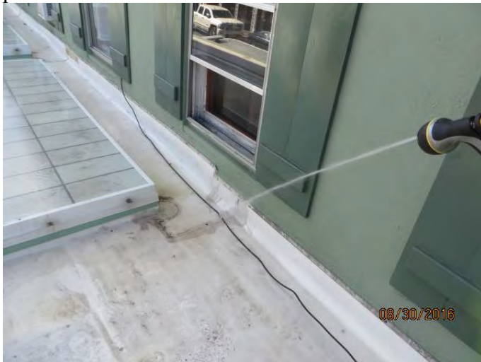
Photo 42 Water test open roof membrane at eighth window from the west shown in photos 31 and 32. Started water test at 10:08 AM
