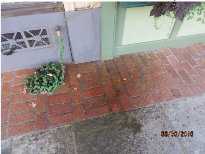
Photo 36 Water on sidewalk beneath leak of photo 35
