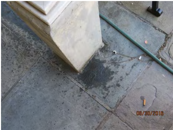
Photo 18 Water on sidewalk from leak Clock Shop sign
