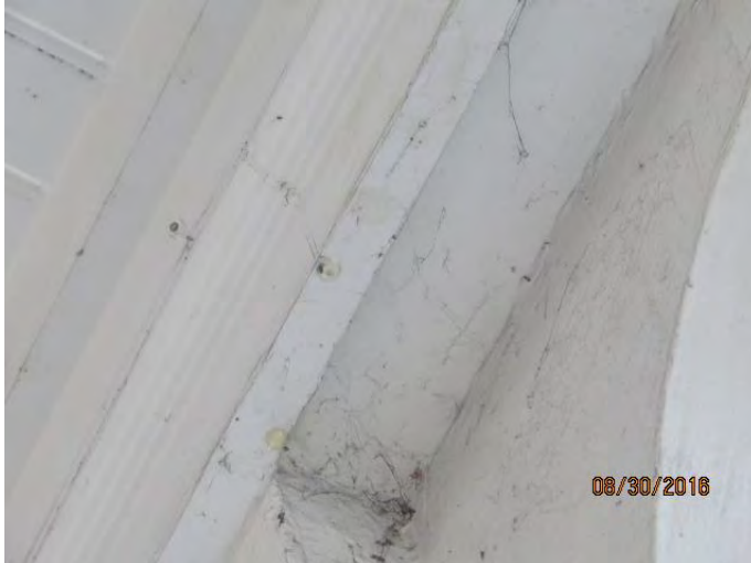
Photo 17 Close up of photo 16, difficult to see water drops
