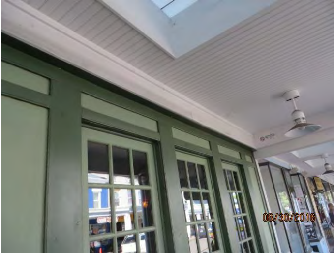
Photo 43 At 10:13 AM water observed at base of white fascia board beneath water test of photo 42
