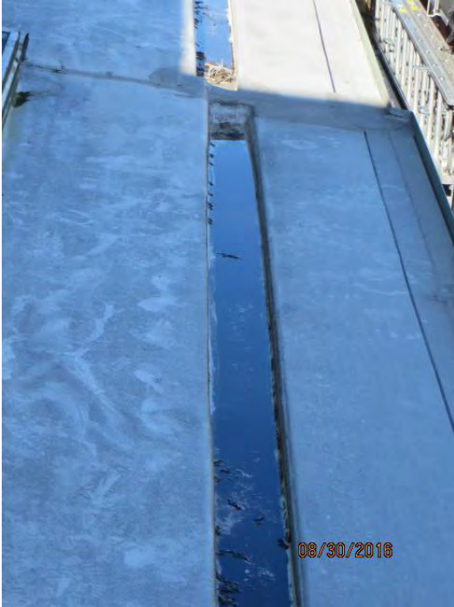
Photo 3 Gutter partially filled
