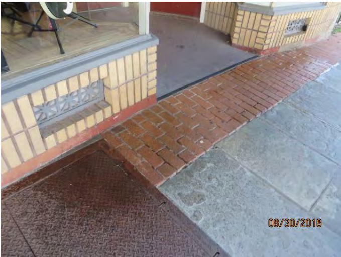
Photo 12 Water on sidewalk across the front of 58 N. Front St.
