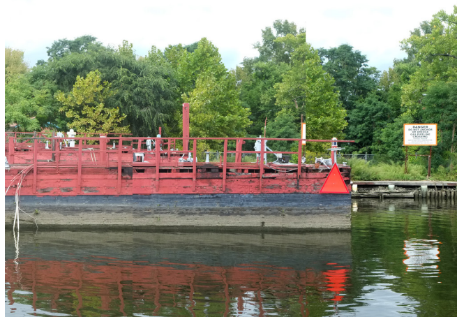
■ ABANDONED DRY DOCK ■ CONCRETE CULVERT GOOD CONDITION
