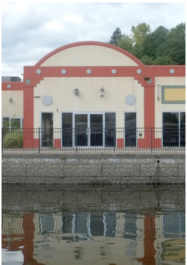
■ STEEL OR CONCRETE BULKHEAD- GOOD CONDITION ■ STEEL OR CONCRETE BULKHEAD- FAIR TO POOR CONDITION
