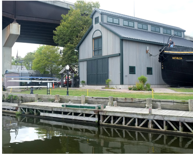
■ TIMBER BULKHEAD- GOOD CONDITION ■ TIMBER BULKHEAD- FAIR TO POOR CONDITION
