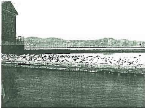
Figure 2 – Kingston-Rondout Lighthouse and Jetty
